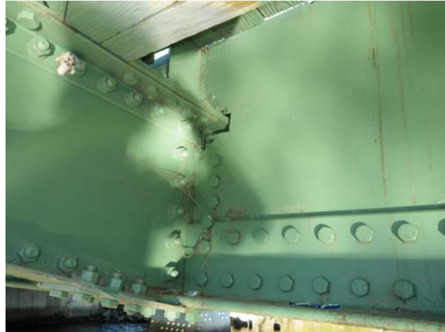
Figure 5: Bracket Connection to Through Girder
