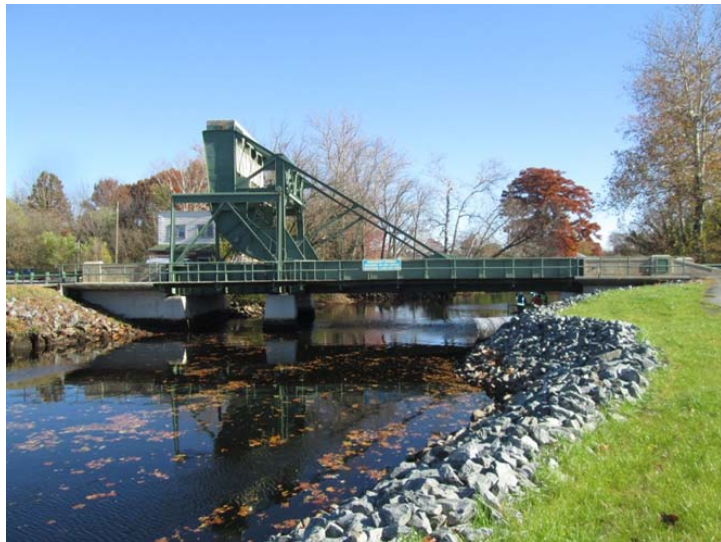
Figure 1: Bridge 3-152 Central Ave. over Broad Creek
