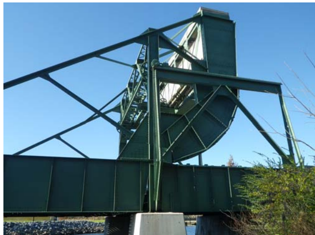
Figure 7: Counterweight, Rack Frame and Segmental Girder
