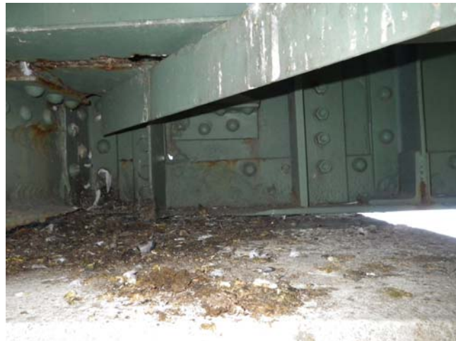
Figure 6: Bottom of West Span 2 Girder at Pier
