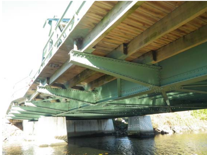
Figure 2: Underside of BR 3-152, looking northeast
