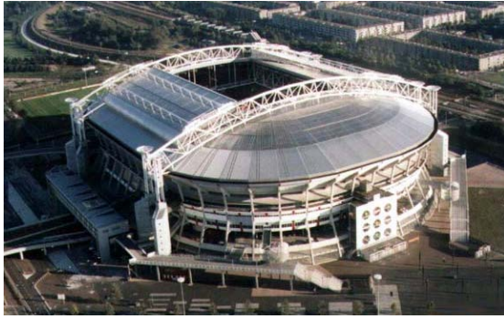
Figure 5: Stiff construction sliding / parallel-, central- movement (Amsterdam Arena, NL, Schalke Arena, Germany) [17]
