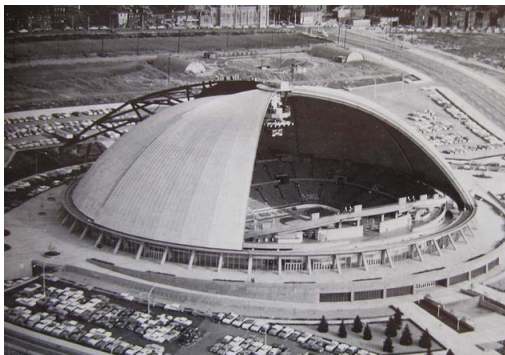
Figure 4: Stiff construction / circular- (Civic Arena, Pittsburgh, US) and Membrane roof / central- movement (Commerzbank Arena, Frankfurt, Germany)
