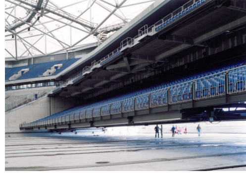
Figure 5: Stiff construction sliding / parallel-, central- movement (Amsterdam Arena, NL, Schalke Arena, Germany) [17]
