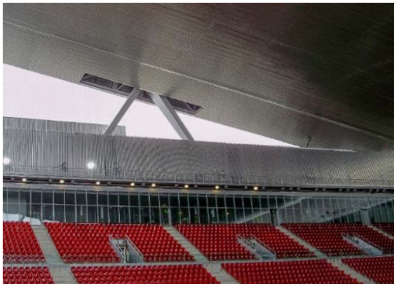
Figure 6: Stiff construction folding central / membrane construction central (Caja Mágica, Spain, Banda Aceh, Indonesia) [17]
