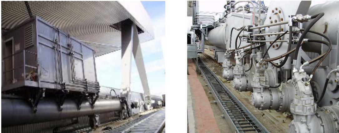
Figure 11: Hydraulic tilting unit with cylinder (left), hydraulic drive system (right) Caja Magica, Spain [17]
