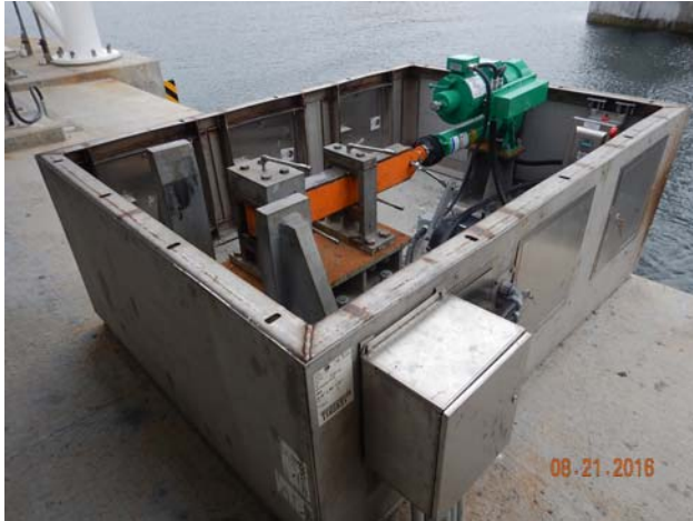
Figure 6: Stainless steel span lock housing (with top cover removed)
