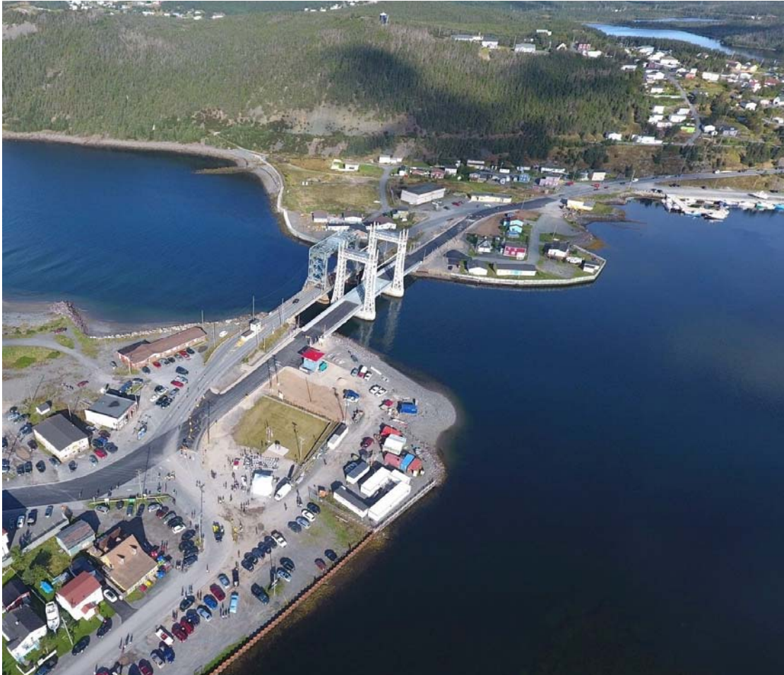
Figure 1: The New Sir Ambrose Shea bridge (right) standing next to the original Sir Ambrose Shea bridge
