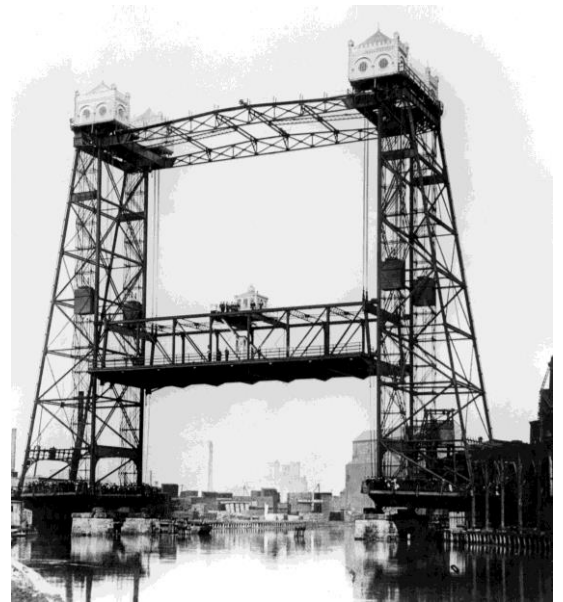
THE HALSTED STREET BRIDGE WAS THE WORLD'S FIRST MODERN VERTICAL LIFT BRIDGE.
