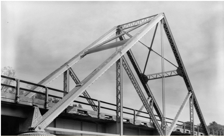
ONE OF TWO SURVIVING EXAMPLES OF A WADDELL "A" TRUSS.
