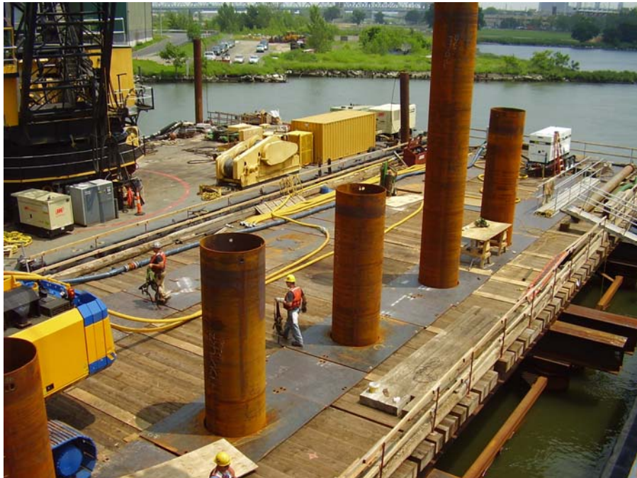
FIGURE 12: Drilled Shaft Installation Platform in Harlem River
