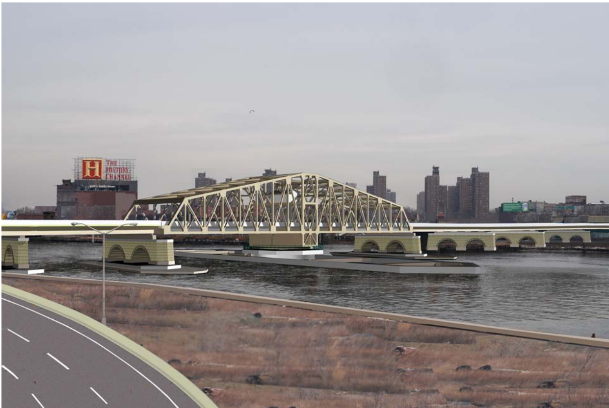
FIGURE 1: New Willis Avenue Bridge
