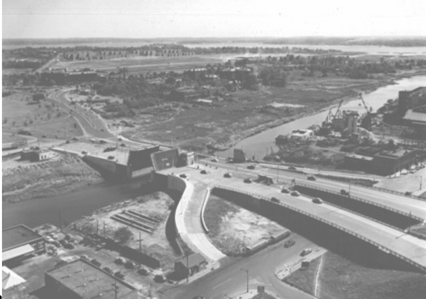
Twin Double Leaf Bascules Prior to Construction of the Expressway
