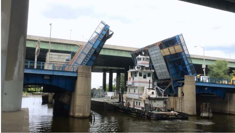
Existing Unionport Bridge
