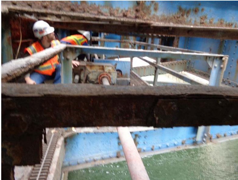
Existing Unionport Bridge confined Machinery spaces
