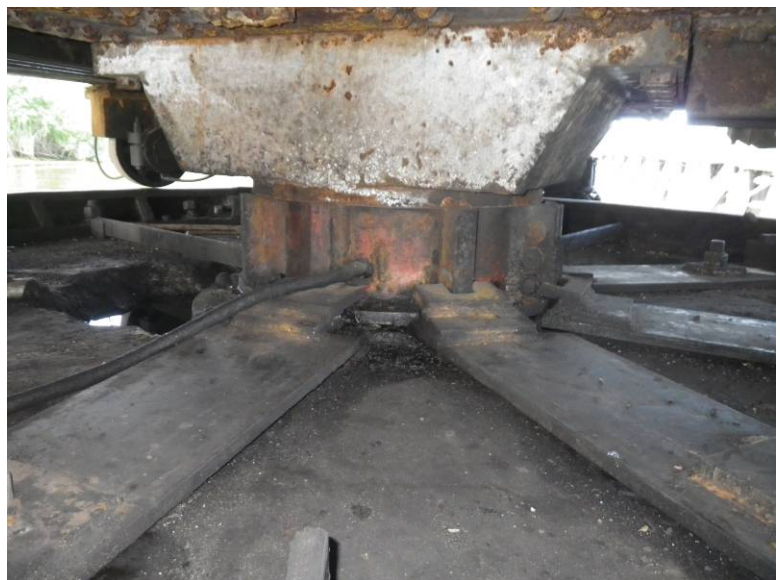
Figure 7. Existing radial struts to secure the rack were connected to the pivot bearing oil box.
