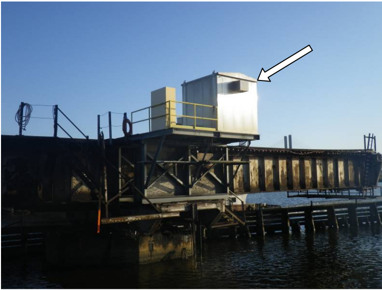
Figure 6. Hydraulic power unit room positioned outboard on the east side of the span.
