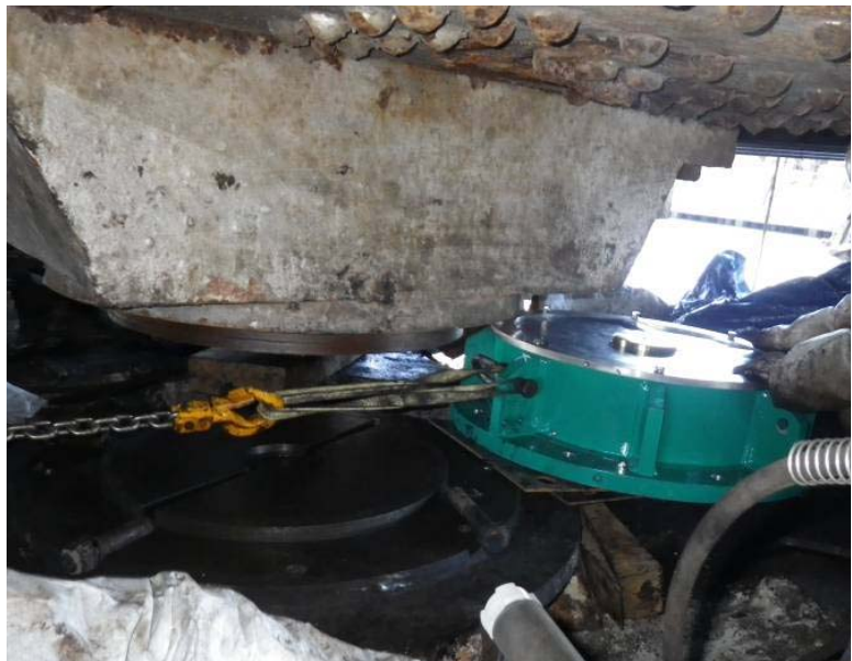
Figure 12. Installation of the new pivot container and bearing disc assembly.
