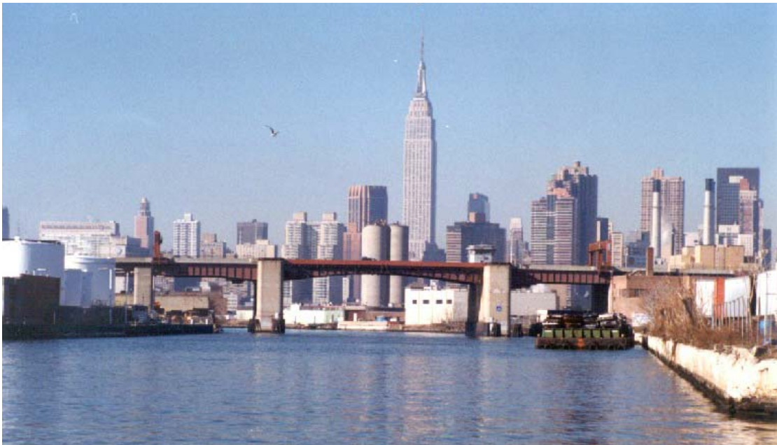
The Pulaski Bridge spans the gateway to Newtown Creek, one of New York City's most important waterways.
