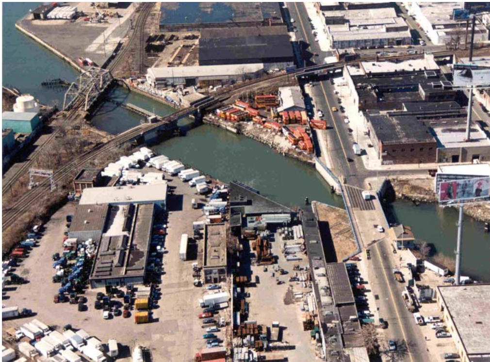
The study took a coordinated approach to multiple bridges on each waterway, including coordination with the Long Island Rail Road regarding its bridges on Dutch Kills.
