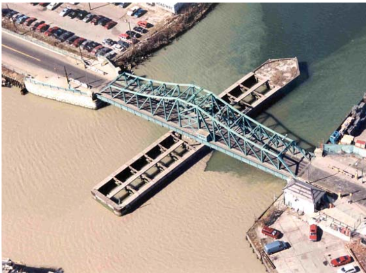
The narrow Grand Street Bridge was identified as a potential candidate for replacement with a fixed bridge.
