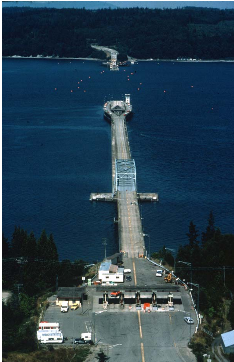
Figure 1 – Aerial Photo Showing Existing East Half (1958 Design) and Sunken West Half.
