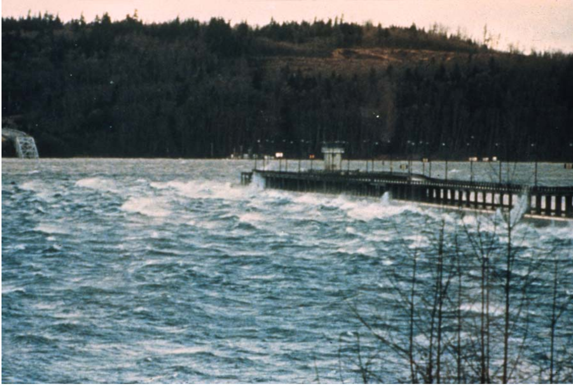
Figure 2 – East Half Sunk During 100 Year Storm
