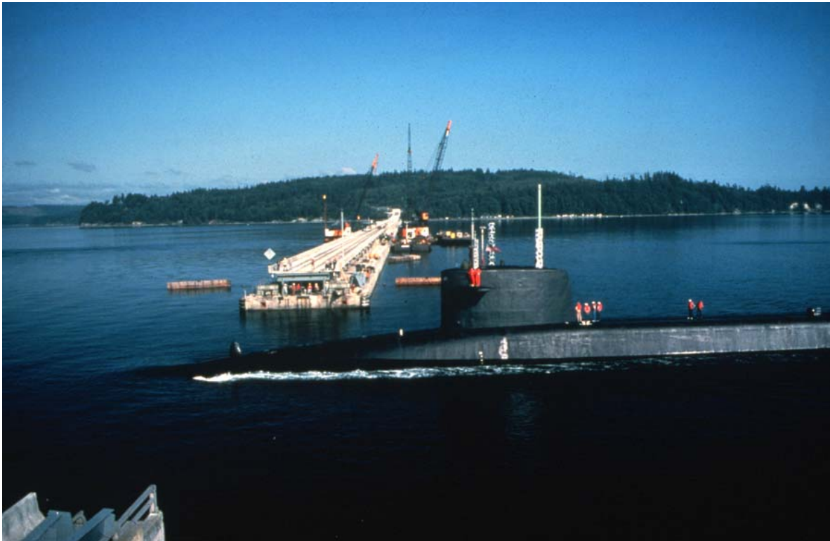
Figure 5 – Submarine Passing Through Open Bridge During Stage I
