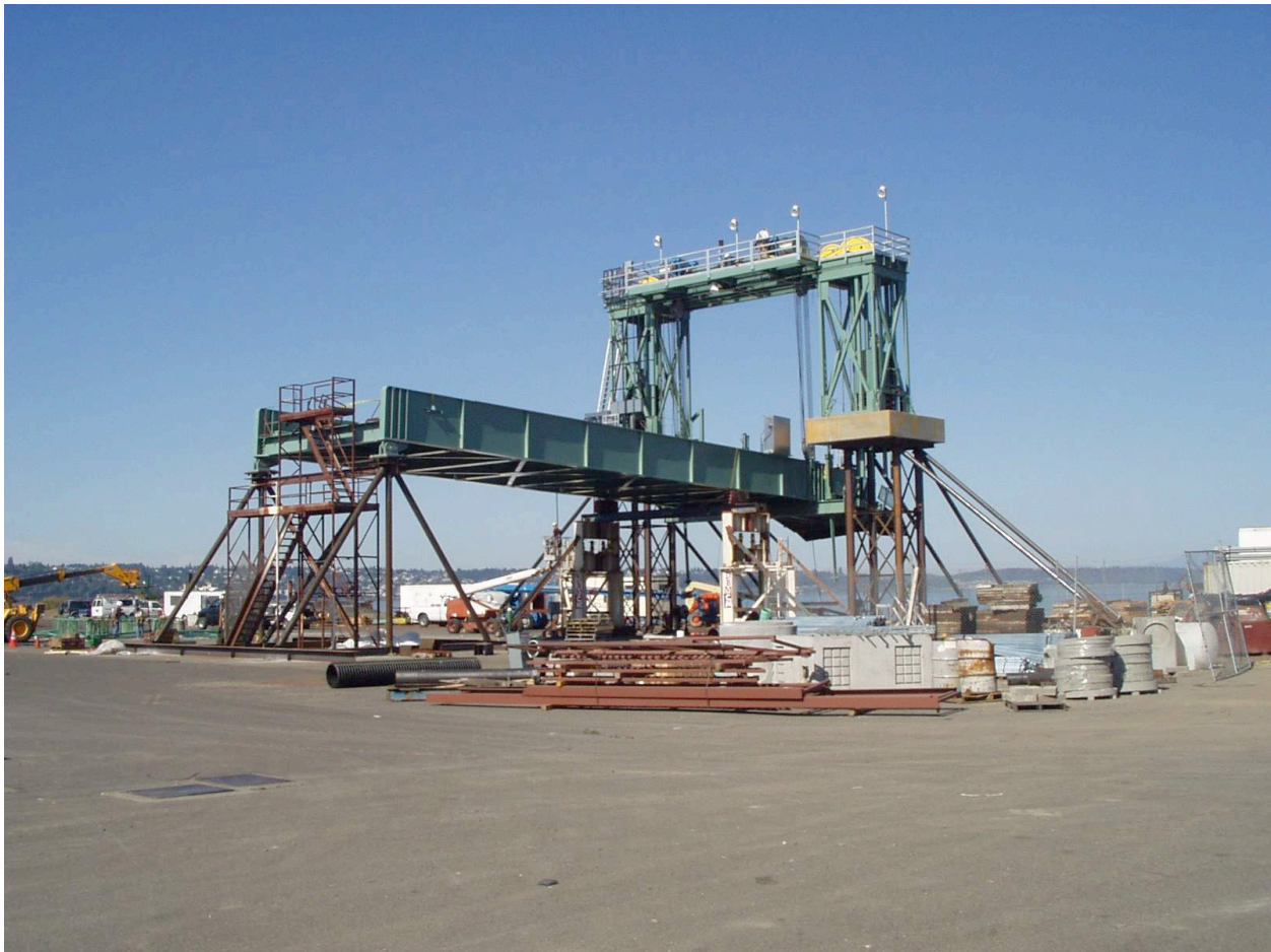
Transfer Span and Lift System during Off-site Construction
