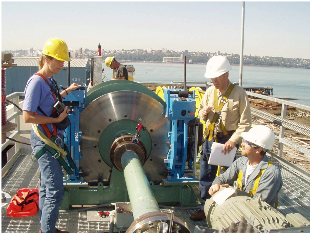
Reducer to Drum Floating shaft being aligned during Off-site Construction
