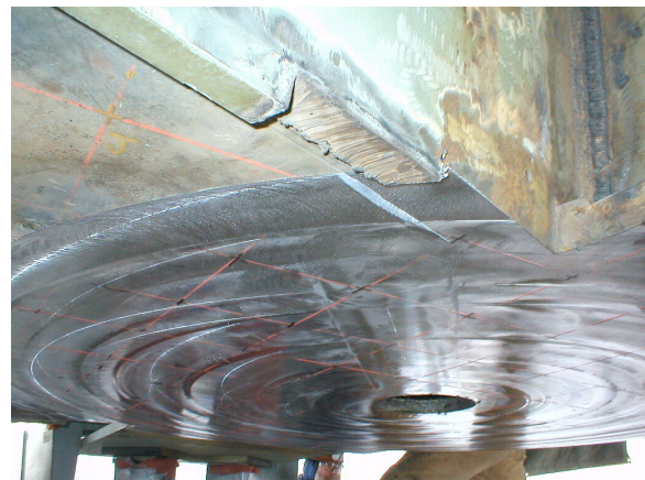
Photo 5: Panel 1L, bottom surface of roof panel after field machining.
