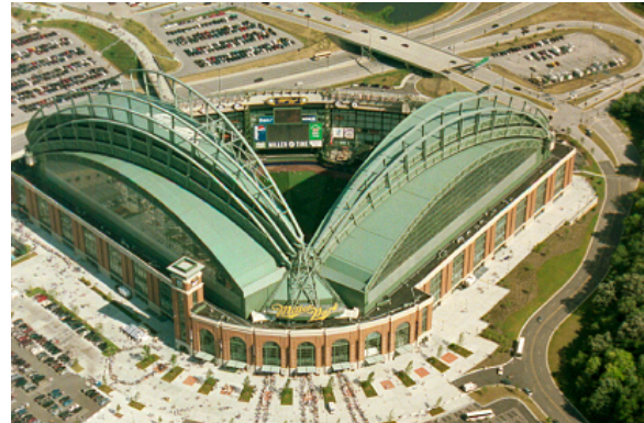
Photo 2: Roof panels shown in the open position.
