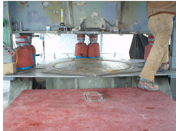
Photo 4: Panel 1, pivot end shown in the raised position after removal of original bearing.
