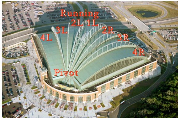
Photo 1: Roof panels shown in the closed position.
