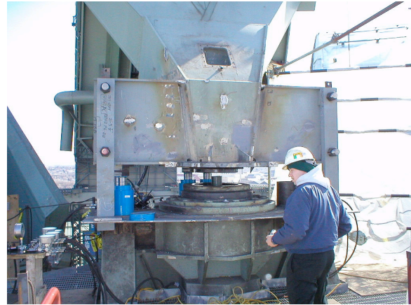
Photo 3: Panel 1L, pivot end shown in the raised position prior to removal of original bearings.
