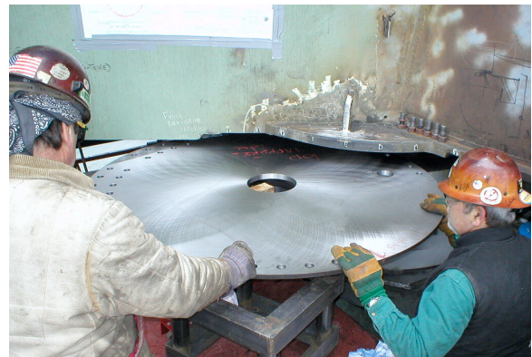
Photo 6: Panel 3L, installation of upper shim plate.
