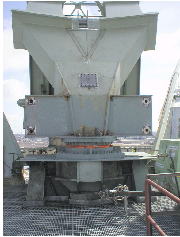
Photo 7: Panel 1L, installation of replacement bearing completed.
