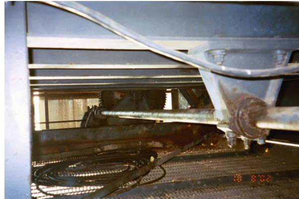
Figure 6: Machinery Area. Note limited space between stringers and grating.
