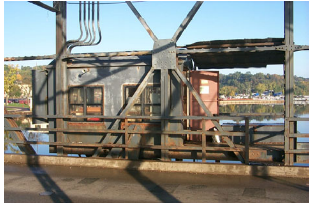
Figure 3: Tender's House. Note chain drive location
