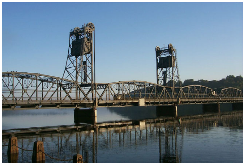
Figure 1: Stillwater Lift Bridge
