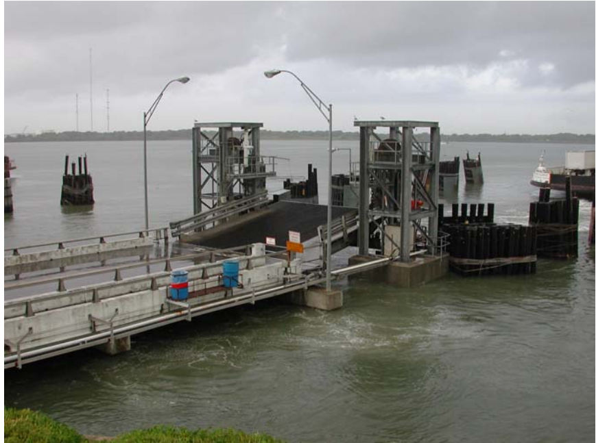
Figure 1. Existing Slip Bolivar-Galveston, Texas.
