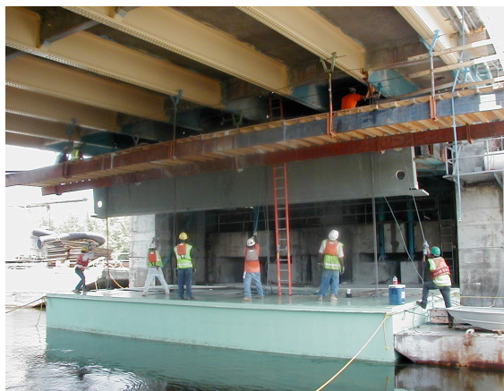
New girder being hoisted into position
