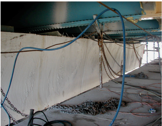
Counterweight concrete condition after saw cut
