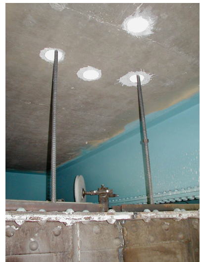
Dywidag bars extending up through flanking
