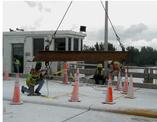
Workers attaching spreader bar and cable rigging to cast eye nuts in preparation to lower counterweight section.
