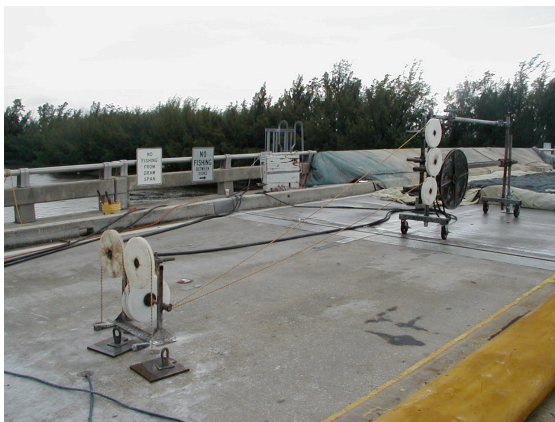
Wire saw pulley system on flanking span. Note support plates and cast eye nut in foreground.
