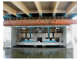
3-way slab completed and first pair of cylinders installed. Second pair is awaiting installation.
