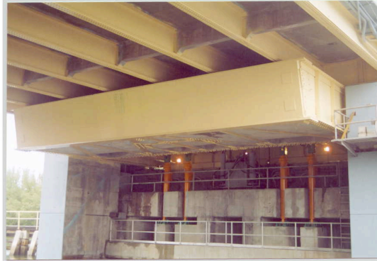
Completed counterweight, machinery area and painting.
