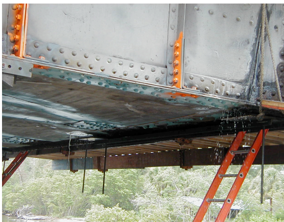
Wire saw making transverse cut through counterweight.
