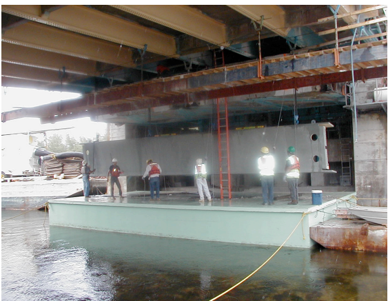
New girder being hoisted into position
