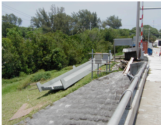
New counterweight girder on-site
