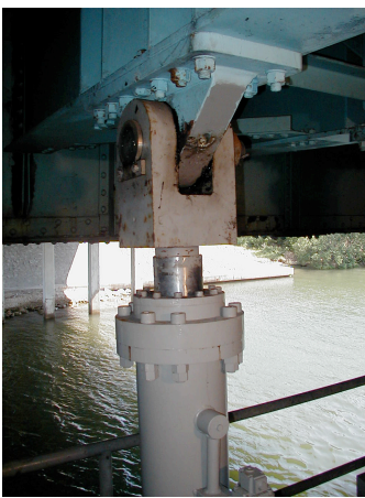
Upper cylinder clevis mount
