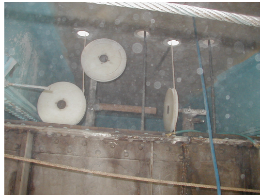
Pulley system beneath flanking span to change wire saw direction
