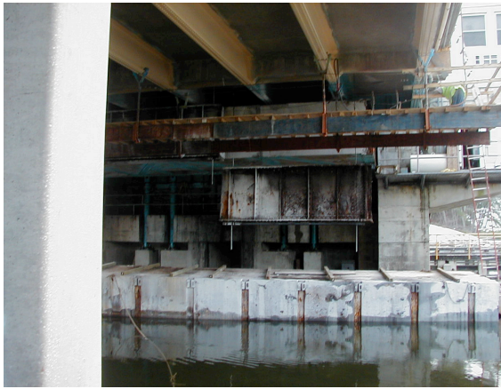
Counterweight section being lowered onto barge.
