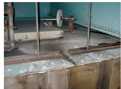
#7 Dywidag bars and channel installed to support counterweight section to be removed.
