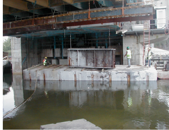
Counterweight section resting on barge.
