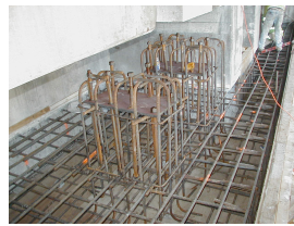
3-way slab and support pedestal reinforcement
