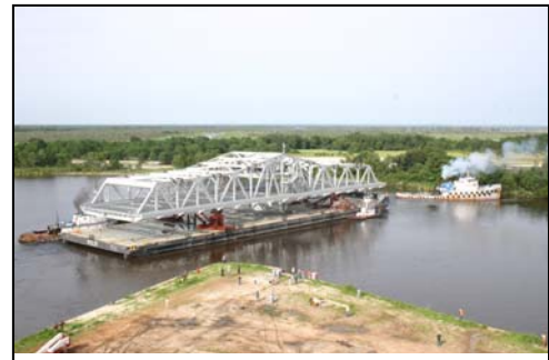
Figure 18: New Swing Span leaving Alabama
