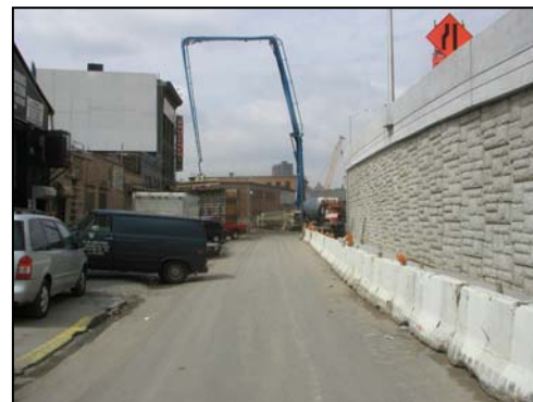
Figure 14: MSES Retaining Wall
