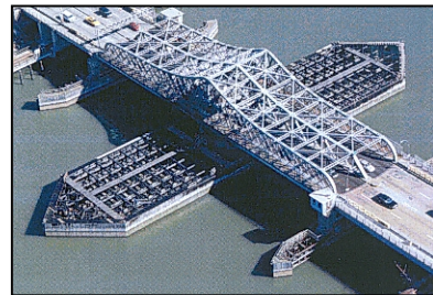
Figure 5: Swing Span of the Third Avenue Bridge
