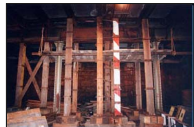
Figure 7: Temporary Shoring supporting the superstructure steel
