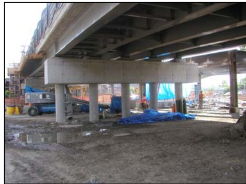
Figure 13: Typical Pier Configuration for the Approach Spans
