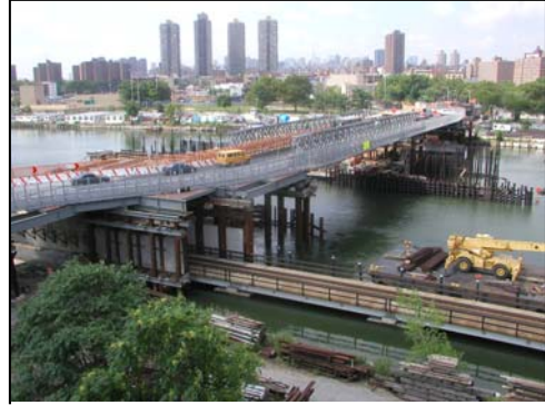
Figure 12: Temporary Bridge over the Harlem River
