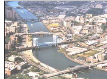
Figure 1: Aerial View of Harlem River Bridges
