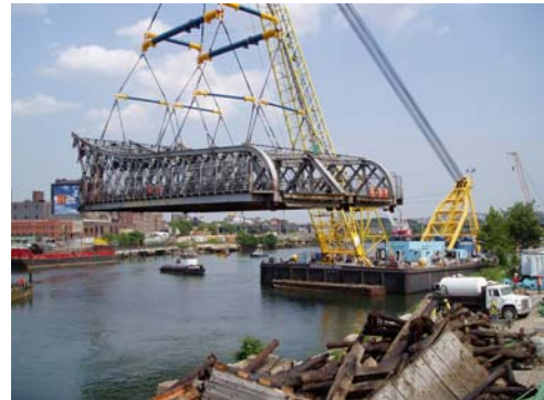
Figure 17: Demolition of Existing Swing Span
