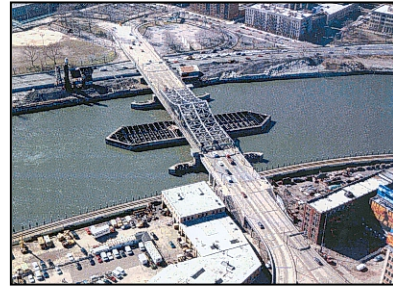
Figure 4: Aerial View of the Third Avenue Bridge
