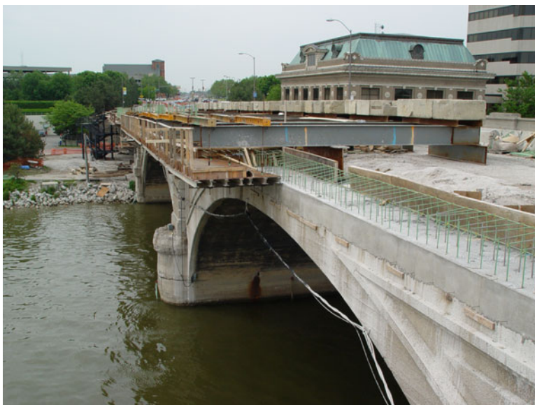
Figure 3 - Arch Span Sidewalk Construction
