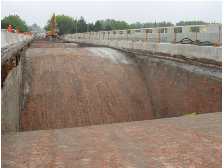
Figure 4 - Arch Spans without Fill
