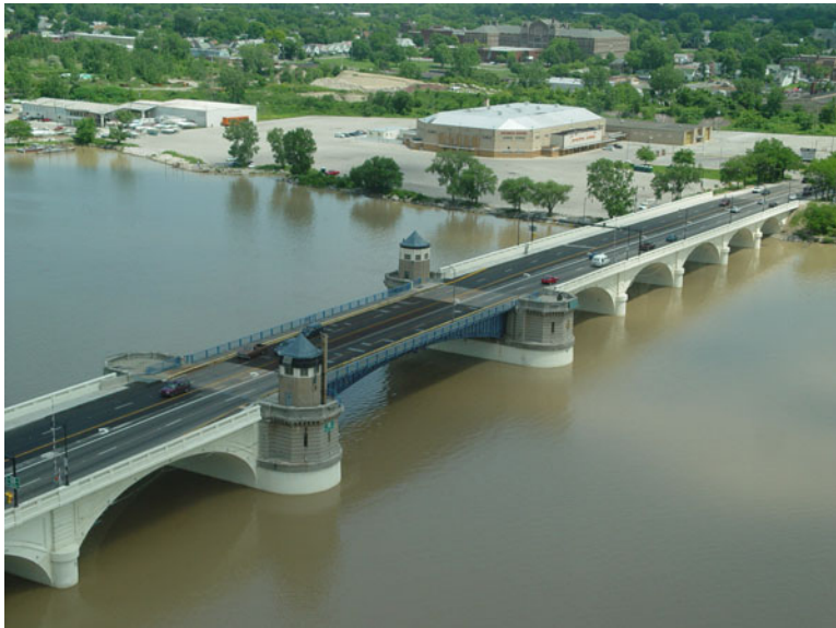
Figure 5 – Completion of Phase 1
