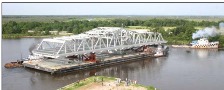
PHOTO 6: Assembled Swing Span Leaving Alabama
