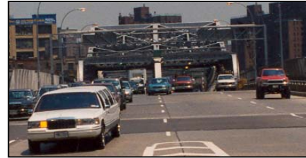
PHOTO 4: Unsafe Weaving Condition (Note Center Truss of Swing Span)
