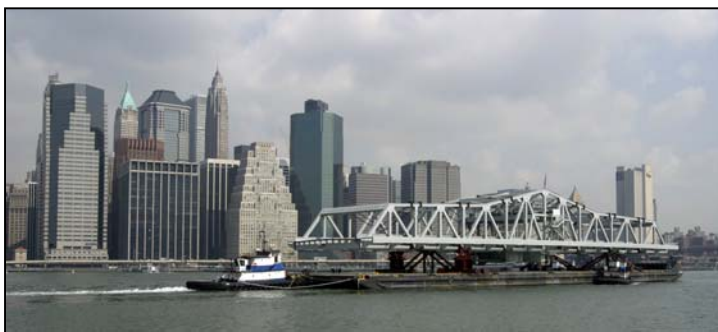
PHOTO 7: Swing Span Passing Downtown New York City
