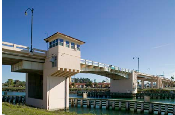
Typical Double-Leaf Bascule Bridge, Venice Avenue, Venice, FL
