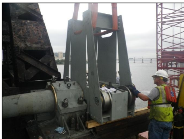
Photograph 9 - View of the top portion of the OSG being installed.
