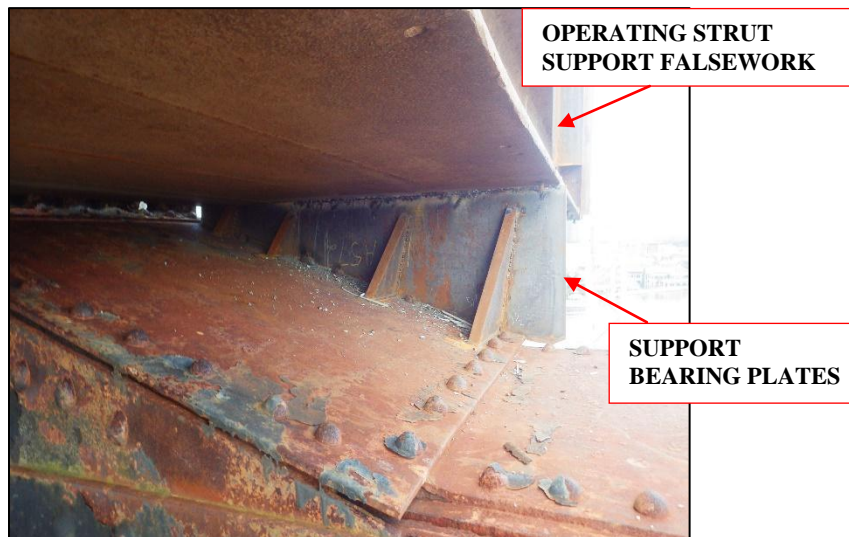
Photograph 4 - View of the bearing plates that were welded to the top of the counterweight truss to support the operating strut falsework
