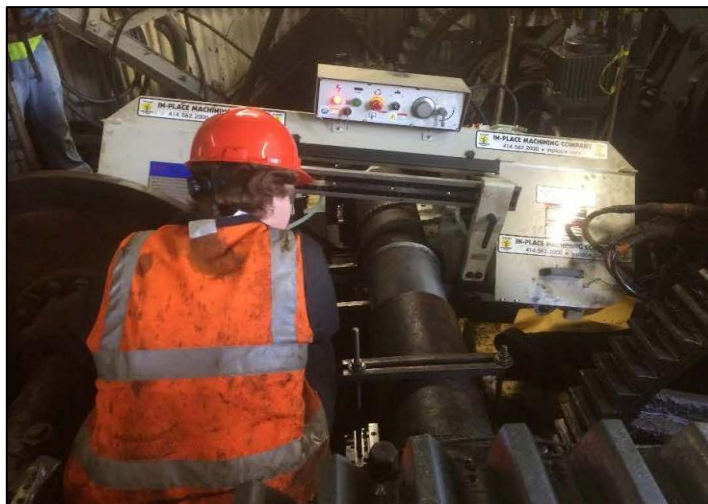
Photograph 17 - View of the 13" band saw cutting the existing cross shaft
