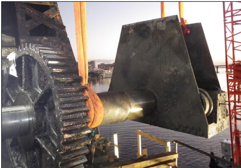
Photograph 8 - View of the existing pinion shaft being removed from the structure. Note that the carriage assembly is being removed at the same time.
