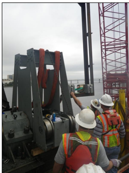
Photograph 10 - C-Hook used to place bearing caps on underside of OSG
