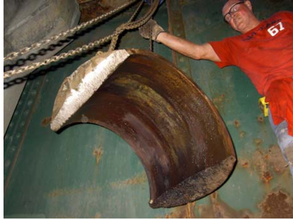
Photo – Old Bearing Removal
