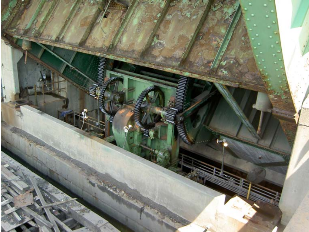
Photo – Span Operation
