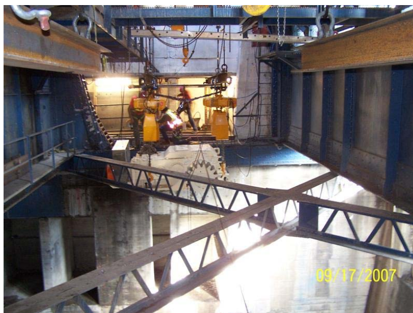
Secondary reducer installation sequence.
