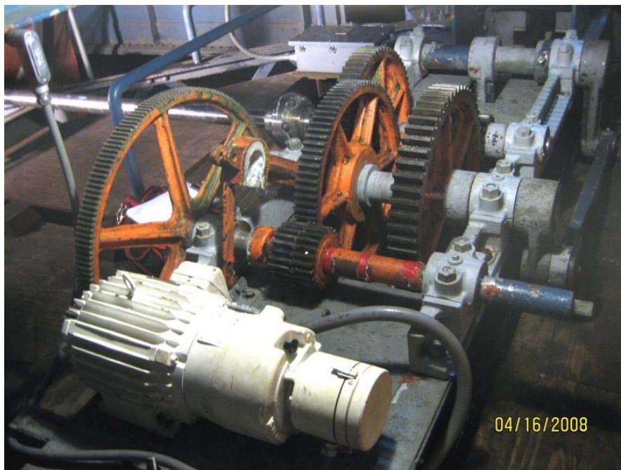
Rehabilitated span lock operating machinery
