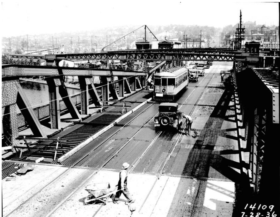
Fremont Bridge, 1936 during re-decking Seattle Municipal Archives Photograph Collection
