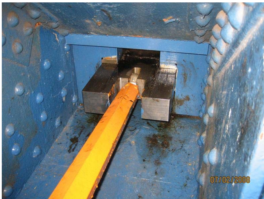
New span lock connecting rod, lock key and guides with bronze wear shoes, shown disengaged.
