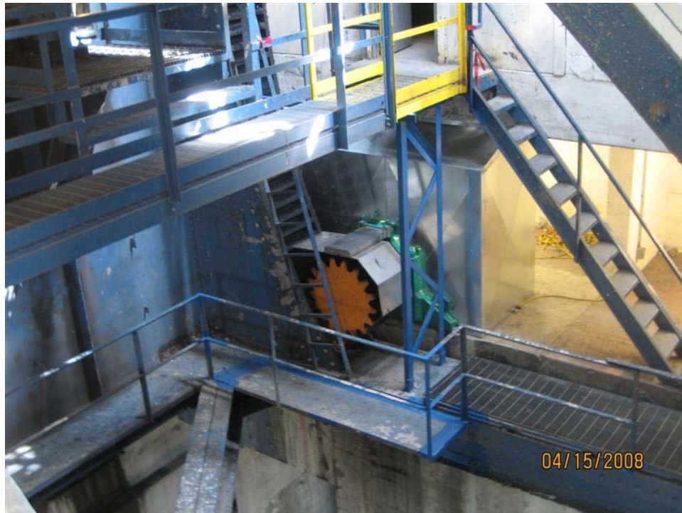
The rack, new pinion and machinery shield viewed from inside the bascule leaf.
