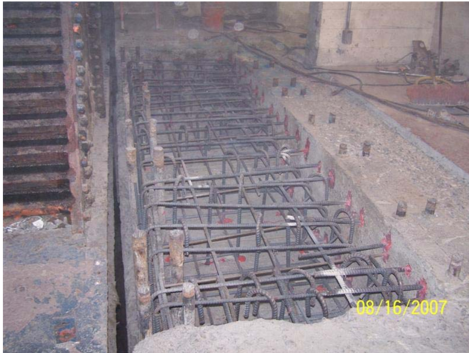
Machinery anchorage modifications.
