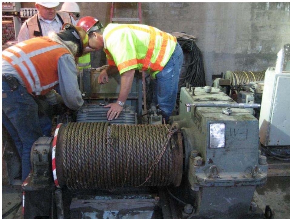
Temporary winch span drive equipment being prepped for installation.
