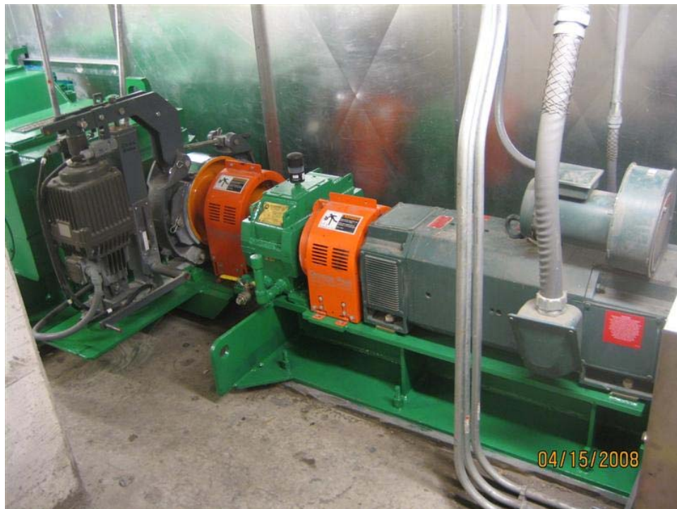
The new span drive motor, primary reducer, motor and machinery brakes viewed from the machinery room.
