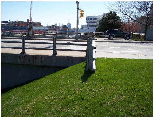
Figure 2: Railing at SW corner of bridge
