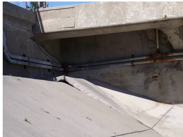
Figure 3: Slope Paving at SE corner of bridge
