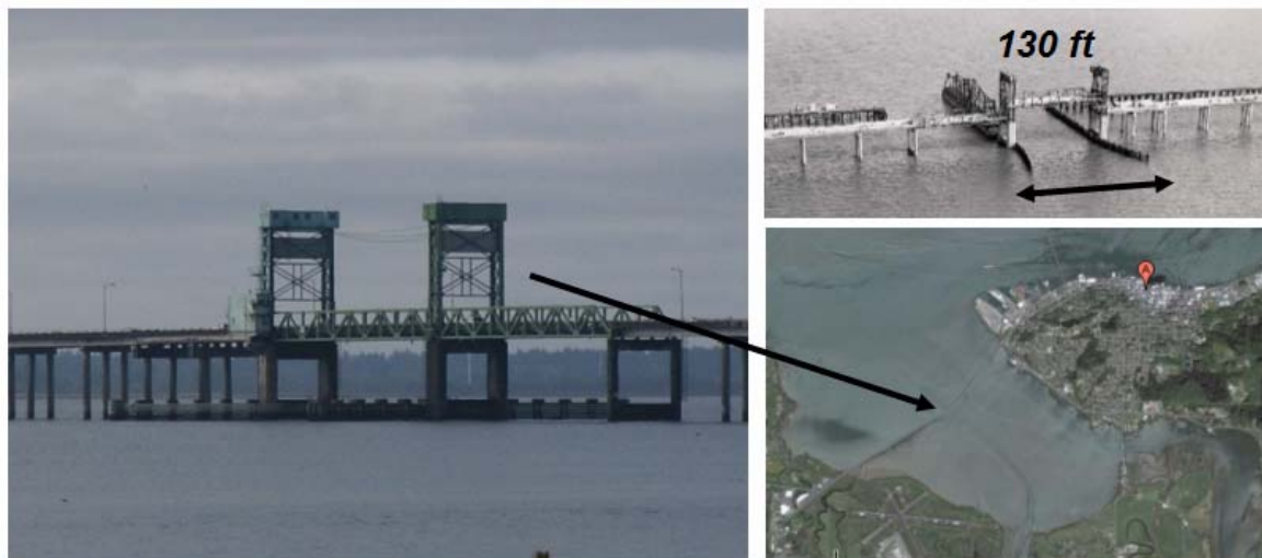
New Young's Bay Bridge (Astoria, OR) combines Optical Rotary Encoder on Near End with Fiber Optic Encoder on Far End (linked via underwater fiber optic cable). Encoders provide velocity feedback to servomotors for synchronizing both ends of lift section.
