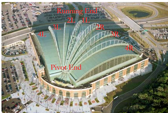
Photo 1: Roof panels shown in the closed position.
