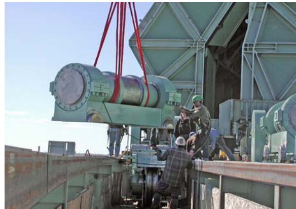
Photo 10: Expansion Assembly being aligned with trucks at track beam level.
