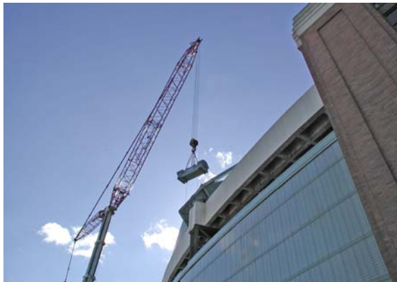
Photo 9: Expansion Assembly being hoisted from plaza level to track beam.
