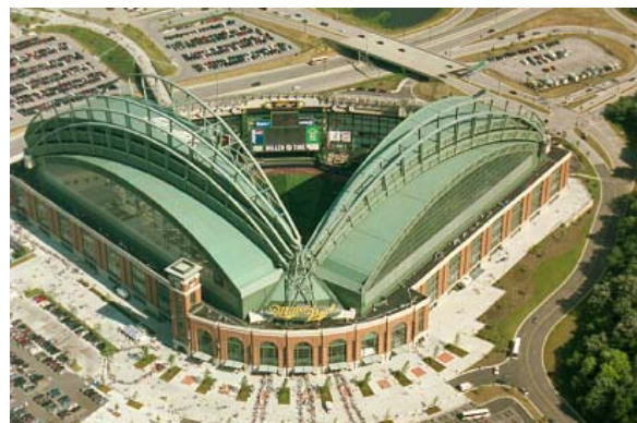
Photo 2: Roof panels shown in the open position.
