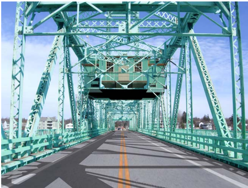
View between the trusses of the new lift span, as designed, showing box and H-shape truss members emulating appearance of built up members on existing span. Note new machinery house above new filled grid roadway.
