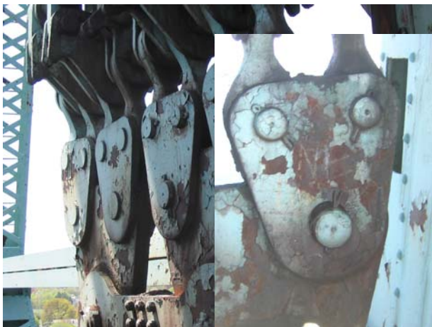
Counterweight rope equalizers. Inset shows worn connection at lower pin.
