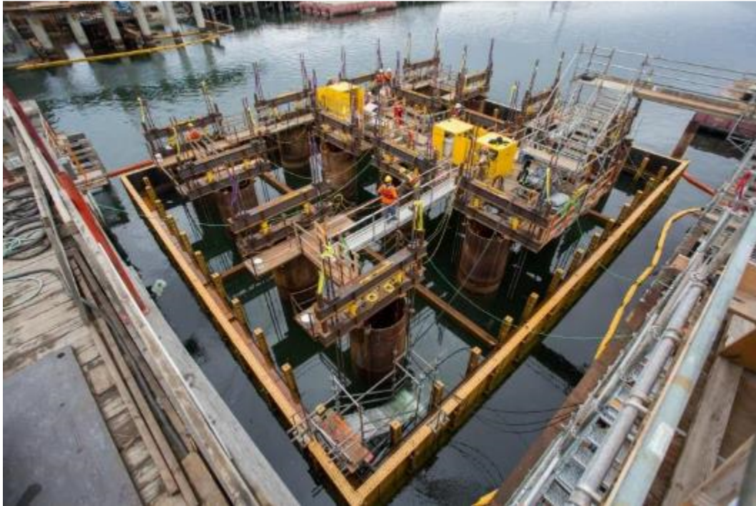
Figure 11: Cofferdam in Lowered Position
