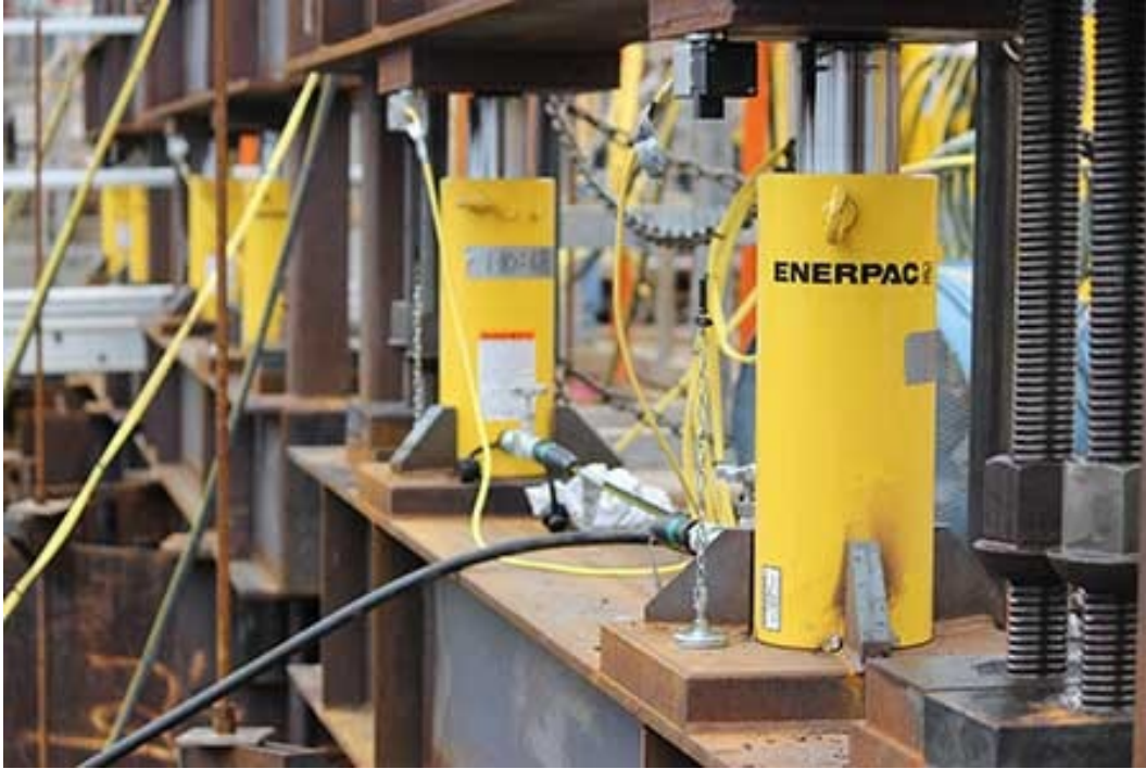
Figure 9: Typical Jack Assembly
