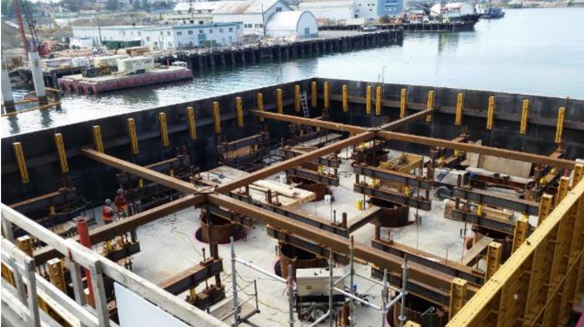
Figure 6: Steel Wall Formwork and Internal Bracing Prior to Lowering
