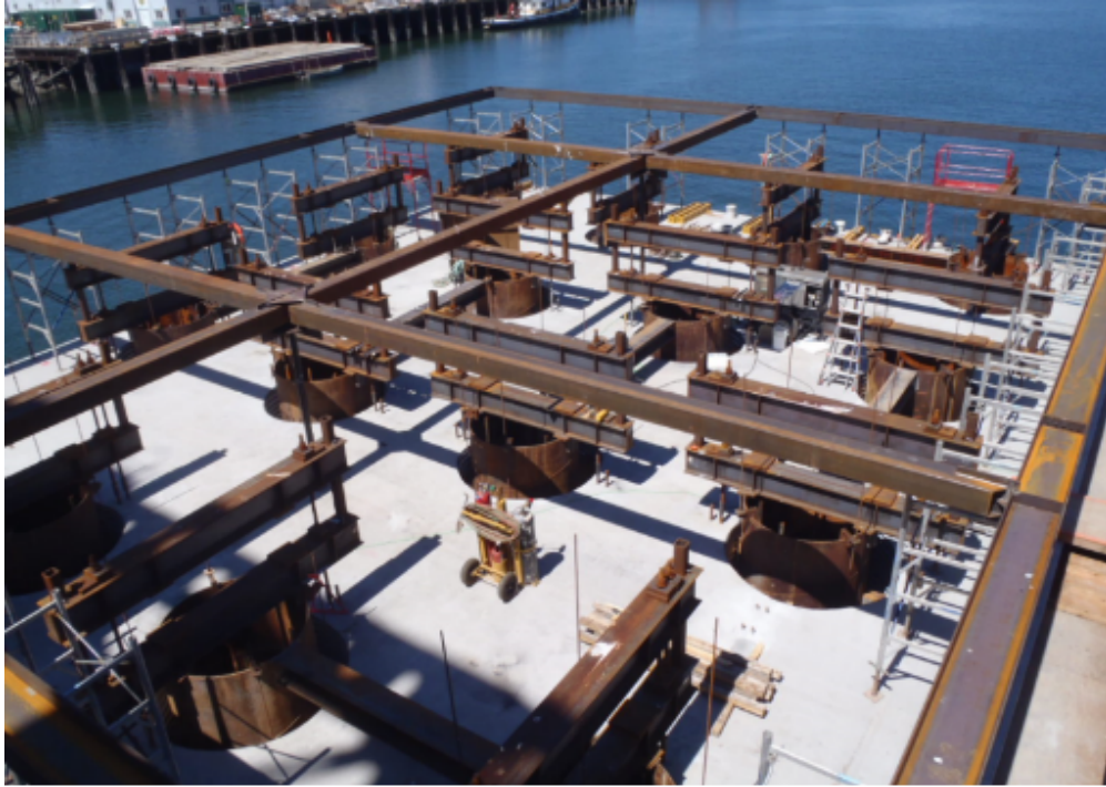
Figure 8: Completed Internal Bracing System
