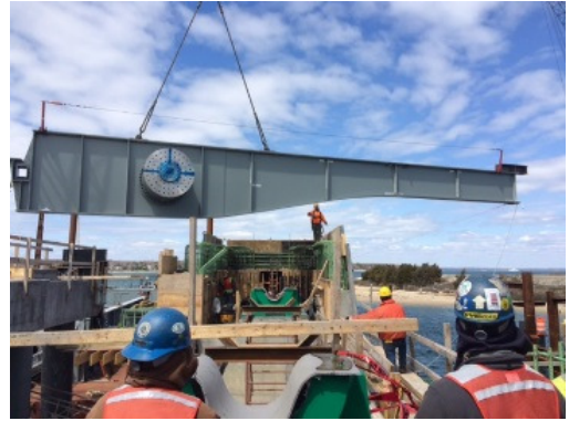
Figure 7: Bascule span lifted into place
