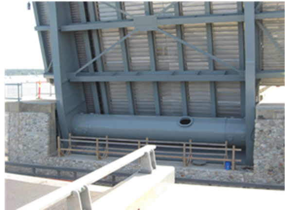
Figure 11: Trunnion Girder between bascule girders visible with leaf in the raised position.
