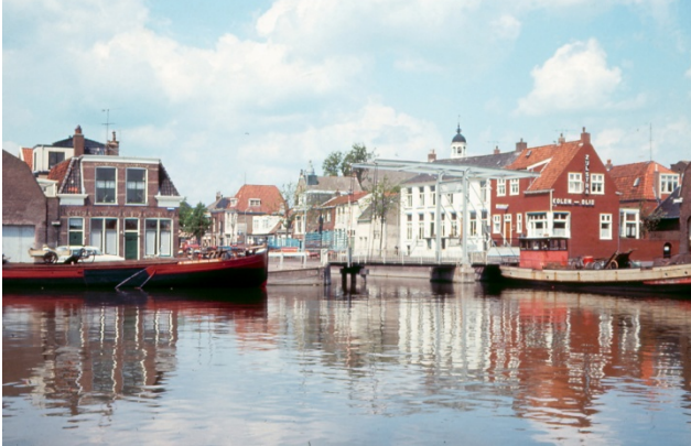
Fig. 1.6: Drawbridge at Kappeln / Netherlands
