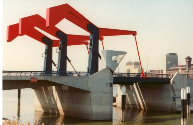
Fig. 1.7: Duffené Bridge at Mannheim
