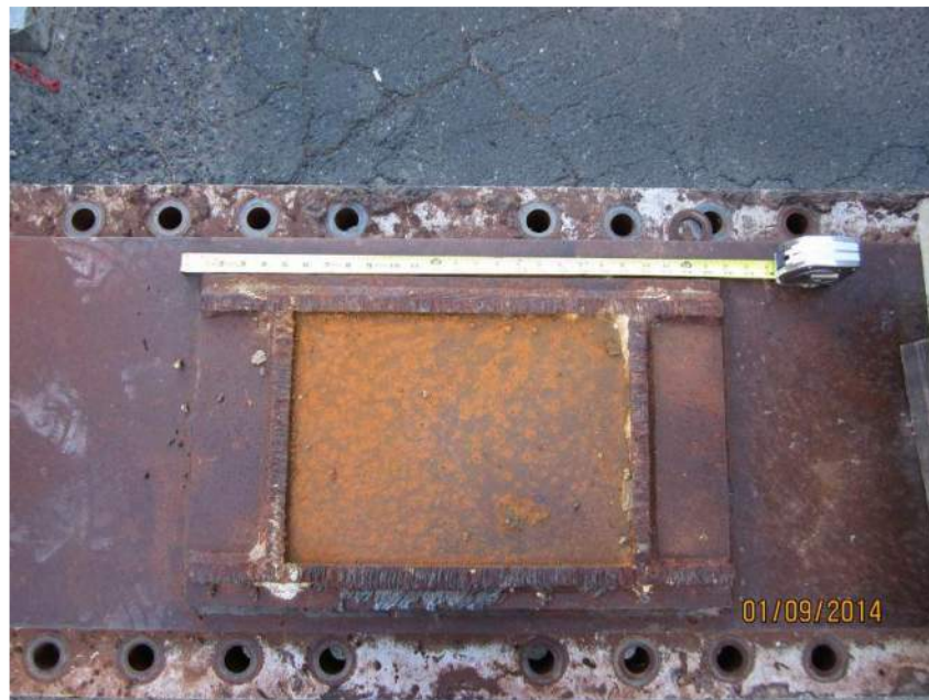
Figure 13 – There is plate welded to the rolling surface of the flat tread that was removed and the surface was repaired.
