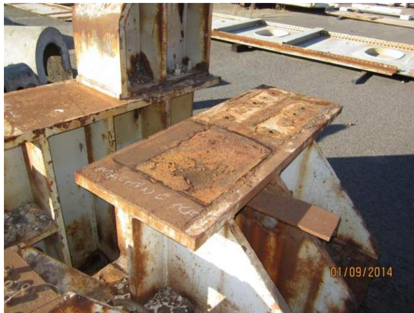
Figure 15 –Live load supports were corroded and were machined to restore a flat surface.
