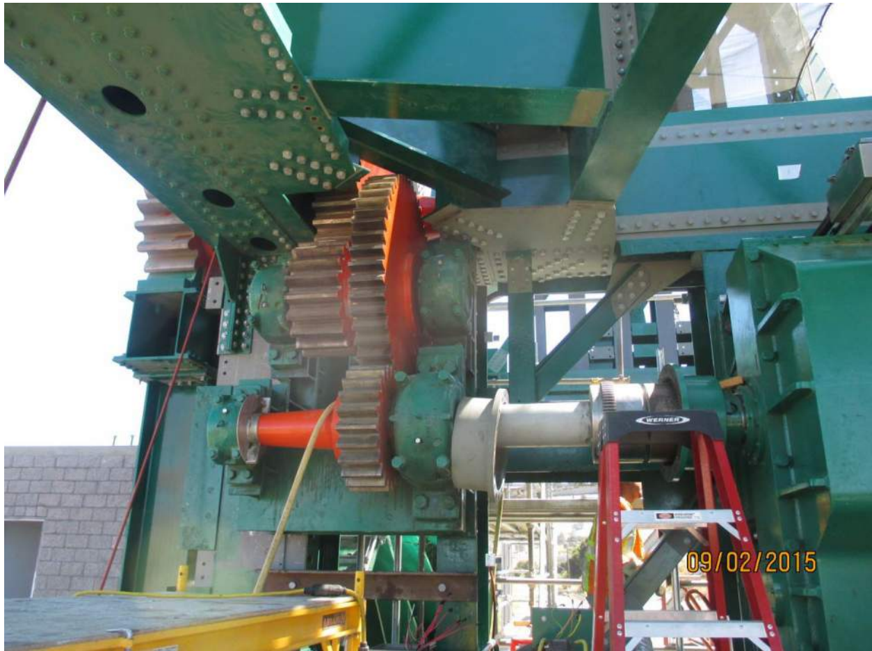
Figure 23 - New Haystack Bridge Span Drive Machinery
