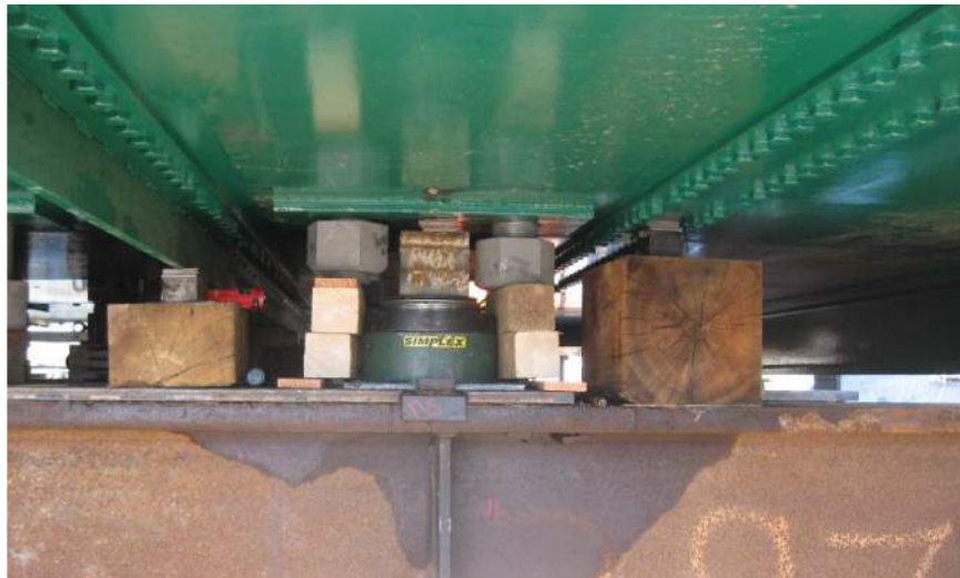
Figure 17 - Counterweight Support Frame
