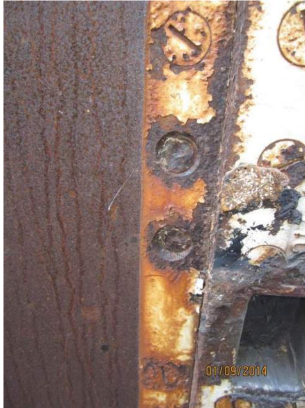
Figure 14 –A few curved tread mounting bolts were found to be damaged or missing and required replacement.
