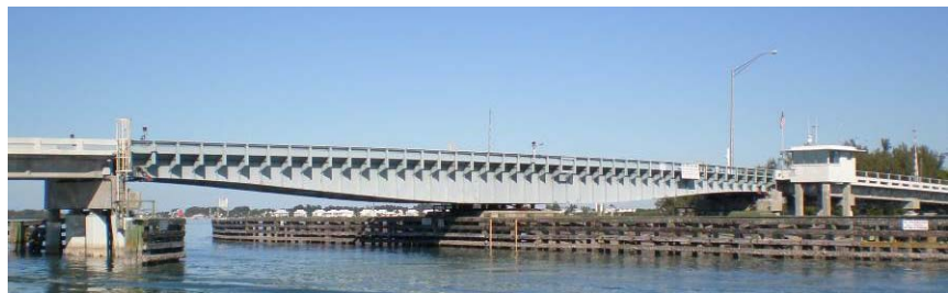
Original Gasparilla Island Swing Span
