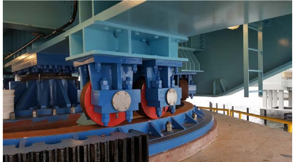
Pivot Bearing and Balance Wheels
