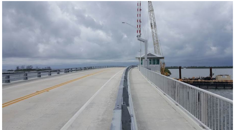
Swing Span Solid Deck
