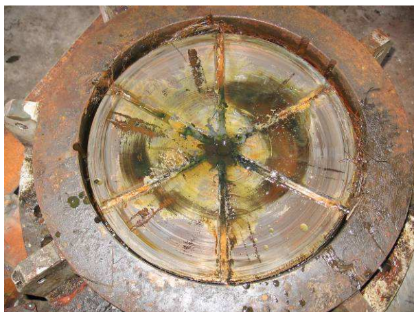
Mermentau River Bridge: Pivot bearing - marsh grass, water, sediment, and rust are visible.
