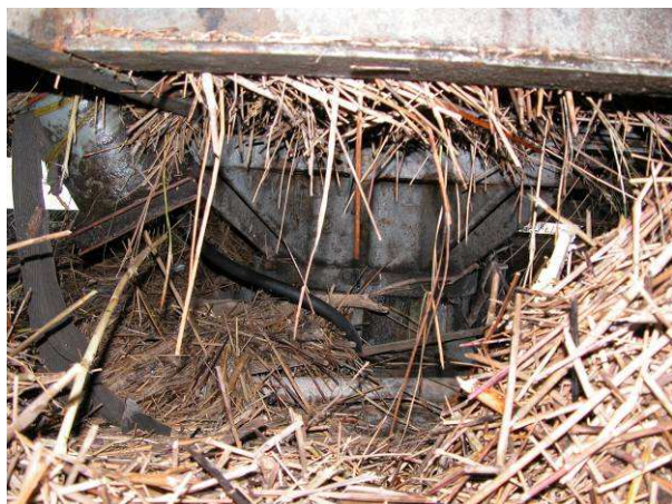
Chef Menteur Pass Bridge: Pivot bearing - obvious evidence of submersion.
