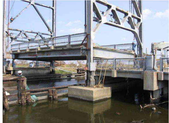
Yscloskey: Span pushed up by storm surge.
