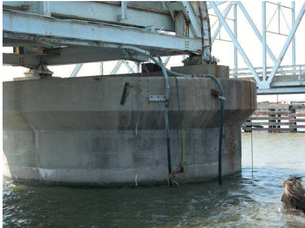
Chef Menteur Pass Bridge: Storm surge current pulled submarine cables from brackets.
