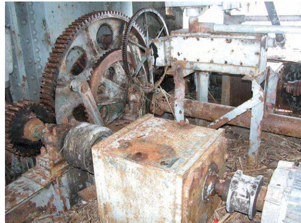
Rigolets Pass Bridge: Submerged gear box
