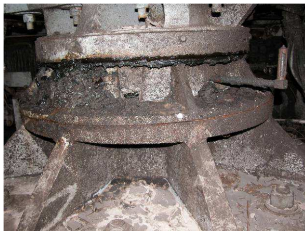
Bayou Bonfouca Bridge: Pivot bearing - obvious evidence of submersion.
