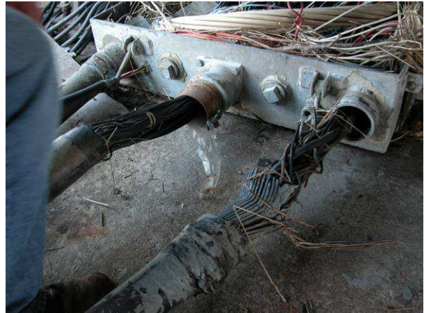
Rigolets Pass Bridge: Storm surge current pulled submarine cables from junction boxes.
