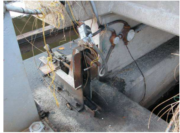
Yscloskey: Span locks tied back.
