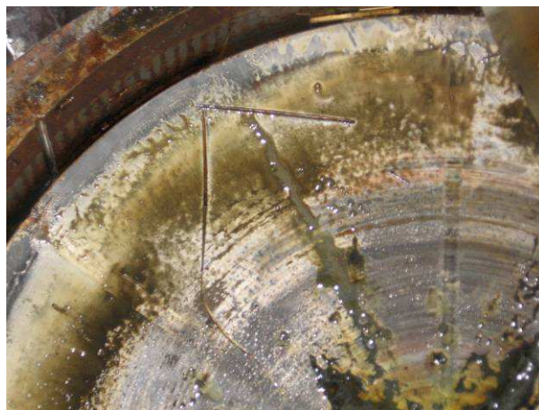
Rigolets Pass Bridge: Pivot bearing - marsh grass, water, sediment, and rust is visible
