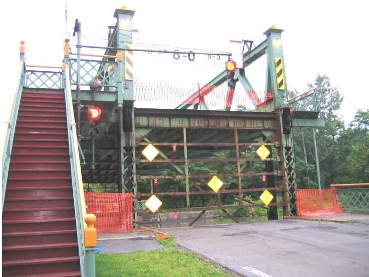
Photo 4: Barrier Gate Integral with Lifting Posts. Note Staircase to Raised Bridge Sidewalk
