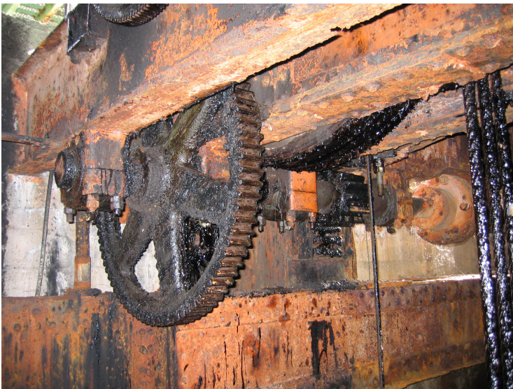
Photo 3: Open gearing and output shaft supported from the counterweight span framing.
