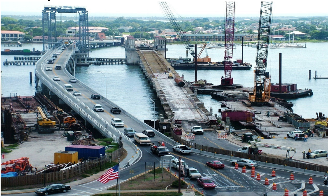
Vertical Lift Structure - Preferred Movable Span Option Opened to Traffic in May, 2006
