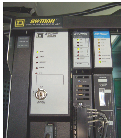
Photograph 3: Square D SyMax Model 500 (Type SCP-523) PLC w/CRM-210 LI Module (Local Interface)
