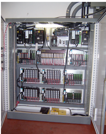
Photo 2: East Structure Control Cabinet
