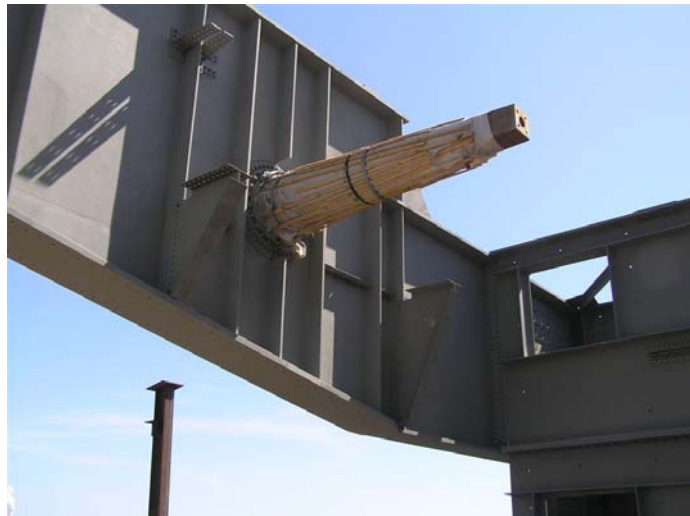
Figure 3 – Bascule Girder with Trunnion Shaft (interior view)
