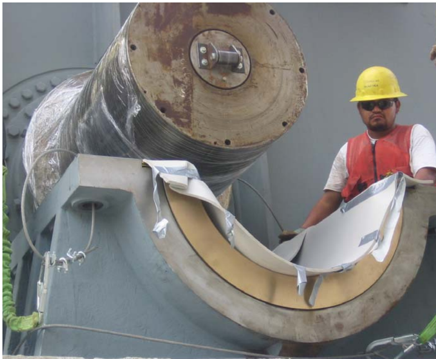
Figure 8 – Trunnion Shaft and Bearing
