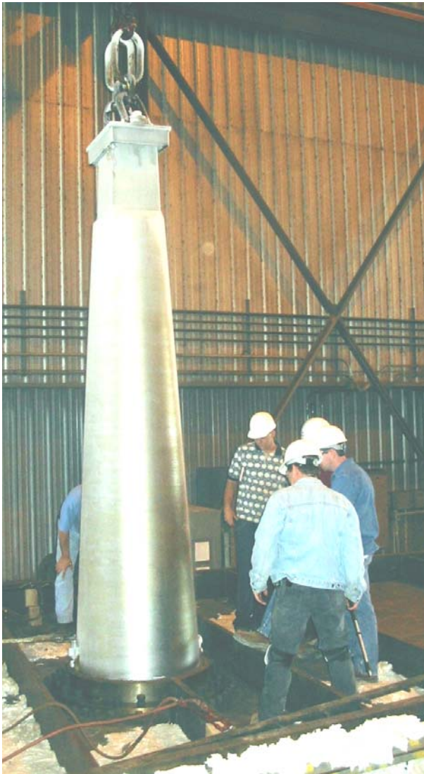
Figure 6 – Fitting the Cooled Trunnion Shaft into the Heated Bascule-Girder Hub
