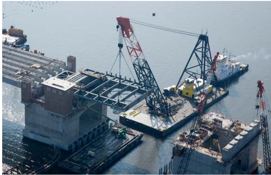
Figure 10 – Erection of East Toe Section
