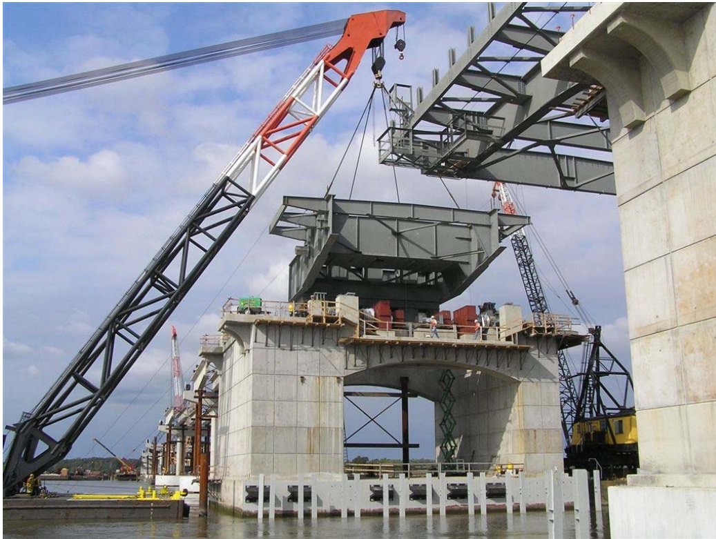
Figure 9 – Erection of West Heel (Counterweight) Section
