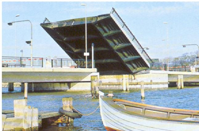
STEKE BASCULE BRIDGE, DENMARK Designed by COWI Civil, Inc. Photo Courtesy of COWI [ FIGURE # 24 ]
