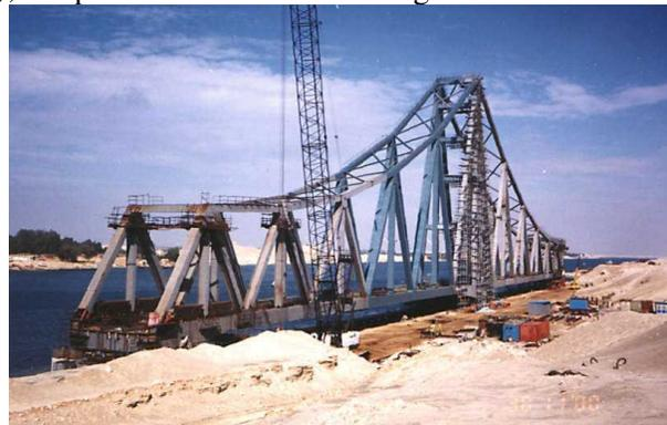
EL FERDAN truss under construction with crawler crane on banks of the Suez Canal 2001. Photo courtesy and by Nick Fuchs PE of Halcrow Group Limited & Egyptian National Railways. [ Figure # 28]
