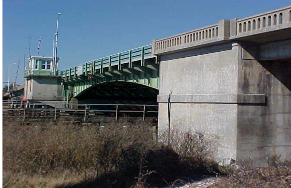
PHOTO 5: General view of Wrightsville Beach Bridge over the Intracoastal Waterway.
