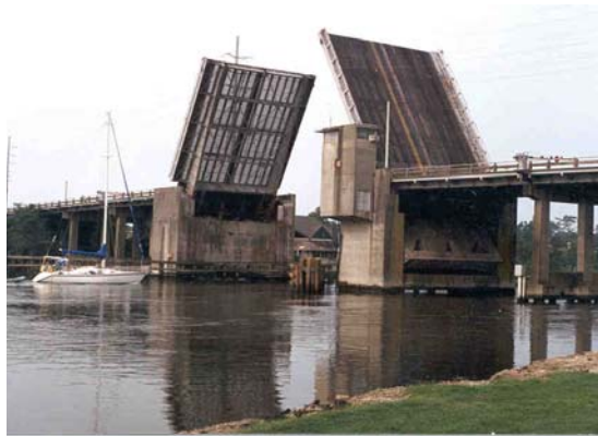
PHOTO 1: General view of Wappoo Creek Bridge prior to reconstruction
