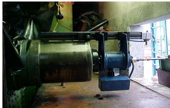
PHOTO 7: Machining system in place on trunnion. Note hole in pier wall to provide clearance.
