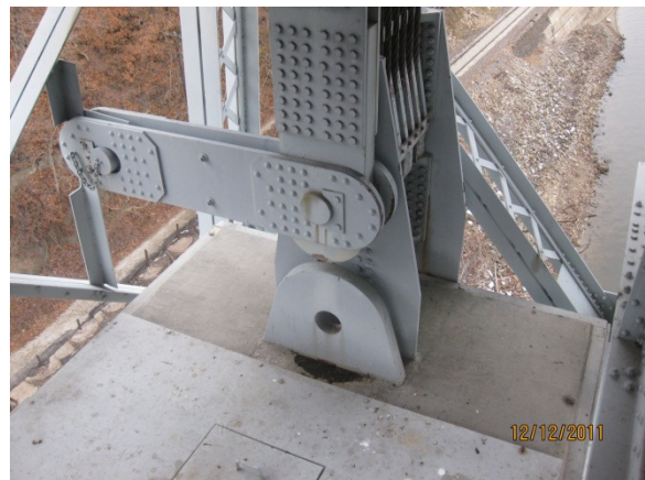
Figure 8. Existing Counterweight Hanger Link in Stowed Position. Lower link is notably longer than distance to clevis connection on counterweight.
