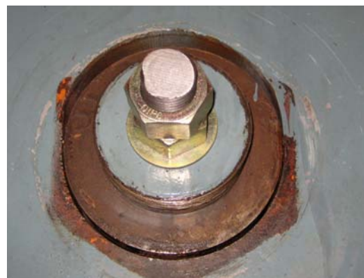
Clearance at underside of Counterweight Pin
