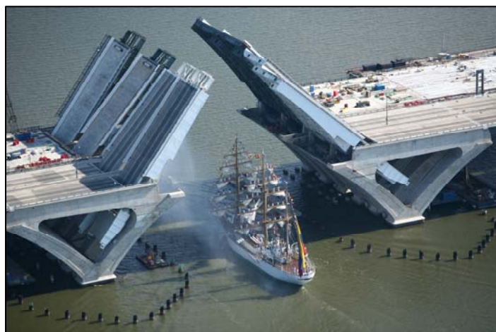
FIGURE 10: New Woodrow Wilson Bascule Bridge in Alexandria, Virginia
