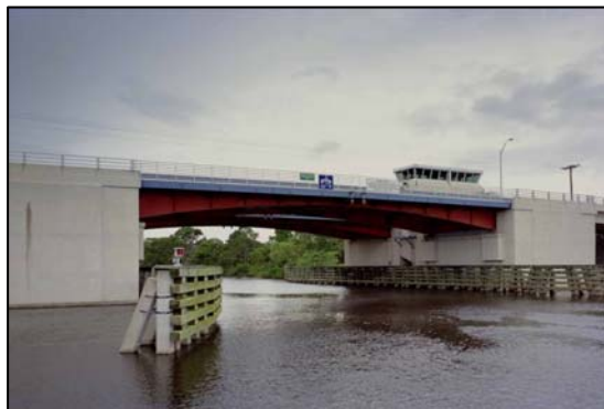
FIGURE 3a: Christa McAuliffe Bascule Bridge - Florida
