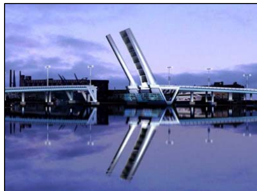
FIGURE 3b: Port River Bascule Bridge – South Australia
