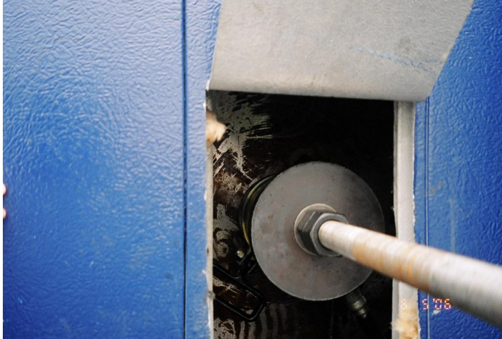
Photo 3: Two Inch Diameter Rod Installed Through Machinery House Wall
