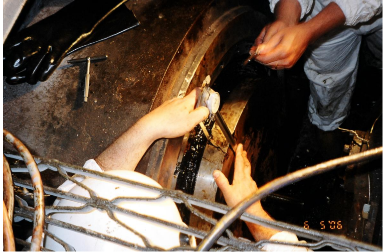
Photo 5: Measurement of Races Prior to Repair Operations
