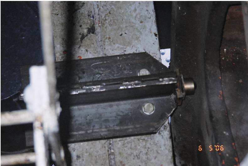
Photo 6: Sheave Guide Roller
