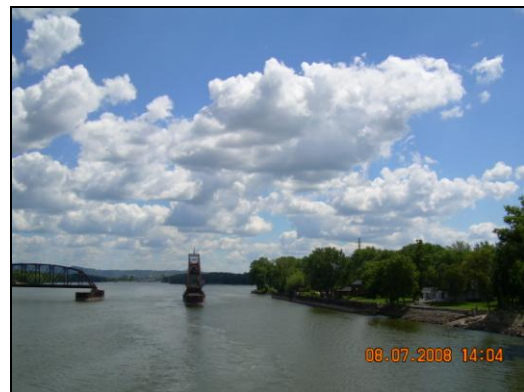
Figure 3 - Existing Swing Span
