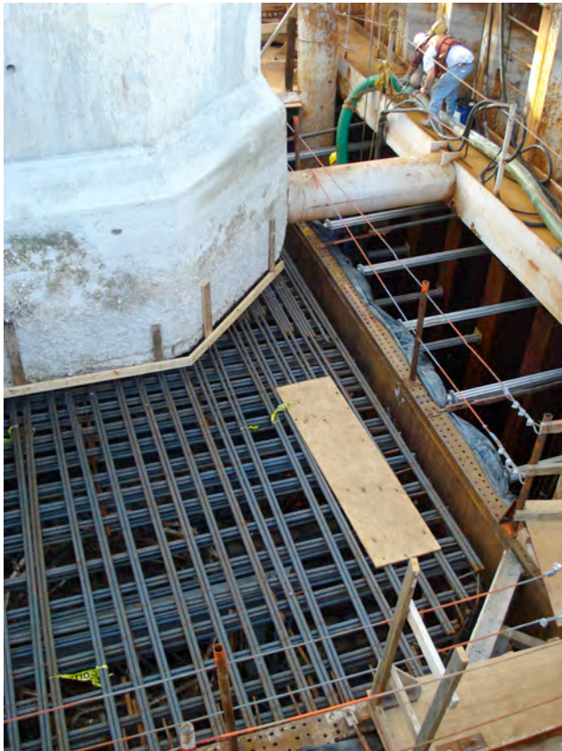
Figure 16 Showing the Top Layer of the Reinforcing Steel in the New Waterline Footing (at a Front/Side Corner of the Pier)
