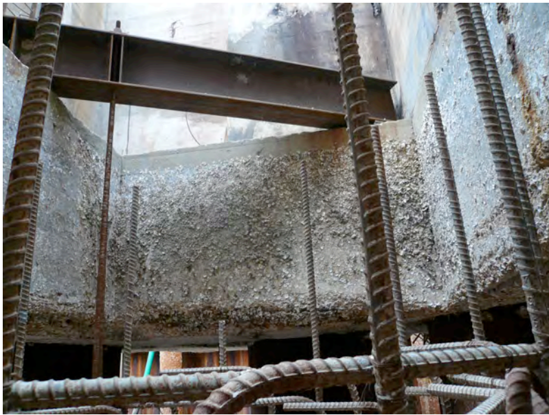
Figure 13 Hangers and Cross Steel Beam for the Falsework at the Opening of the Existing Waterline Footing
