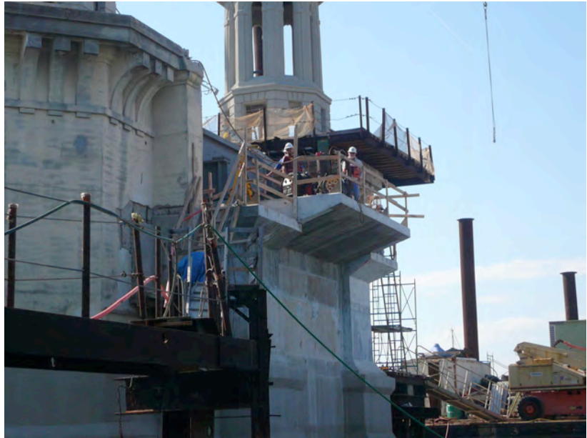
Figure 20 New Machinery Platform Cantilevered from the Existing 18" Wide Backwall
