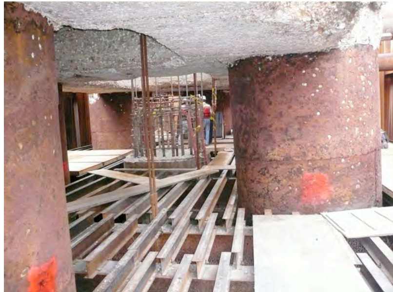
Figure 12 Another View of Falsework under the Existing Waterline Footing
