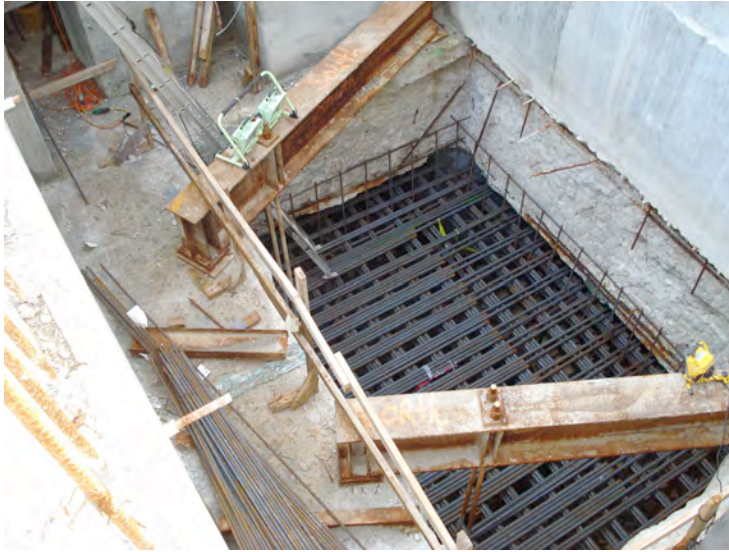
Figure 17 Showing the Top Layer of the Reinforcing Steel in the New Waterline Footing (At the Middle Opening of the Existing Waterline Footing)
