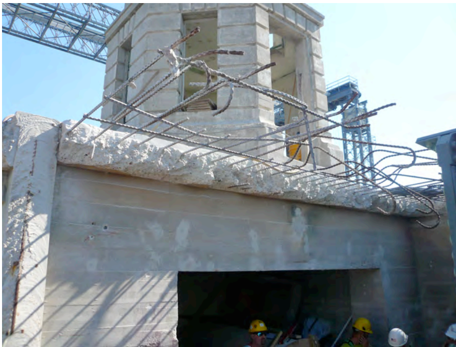
Figure 22 Much Less Than Expected Reinforcing Steel in the Existing Deck
