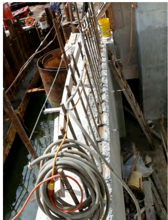
Figure 21 Additional Reinforcing Steel Added by Removing the Back Face of the Backwall
