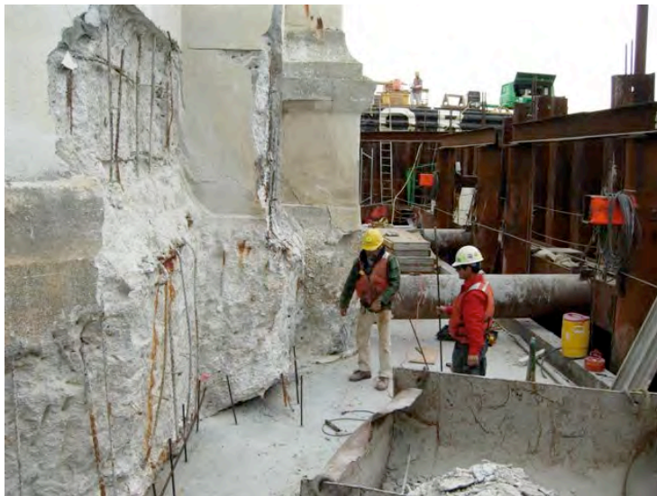
Figure 18 Showing the Newly Poured Waterline Footing and Preparation for Restoring the Existing Bascule Pier Surface
