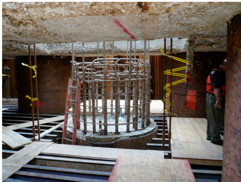
Figure 14 Showing the Falsework Platform at the Middle Opening of the Existing Waterline Footing and the New Drilled Shaft
