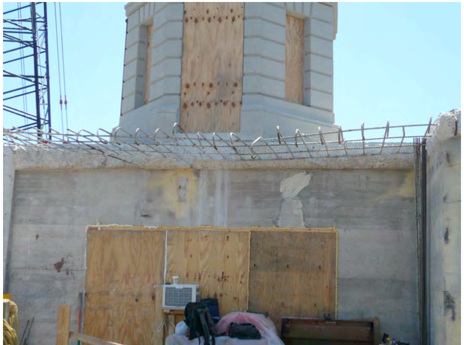
Figure 22 Much Less Than Expected Reinforcing Steel in the Existing Deck
