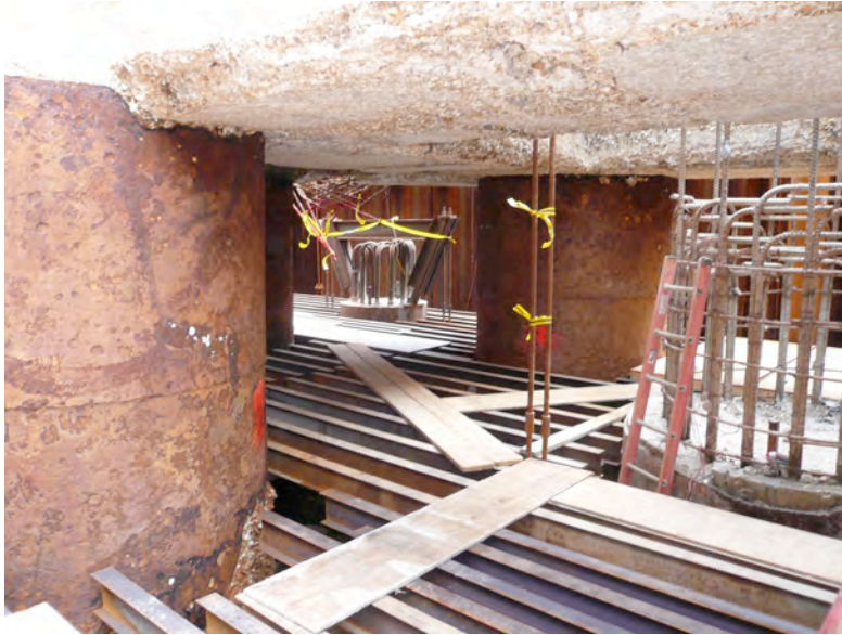
Figure 11 Partial View of Falsework under the Existing Waterline Footing
