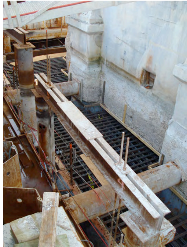
Figure 15 Showing the Top Layer of the Reinforcing Steel in the New Waterline Footing (Back Side of the Pier)
