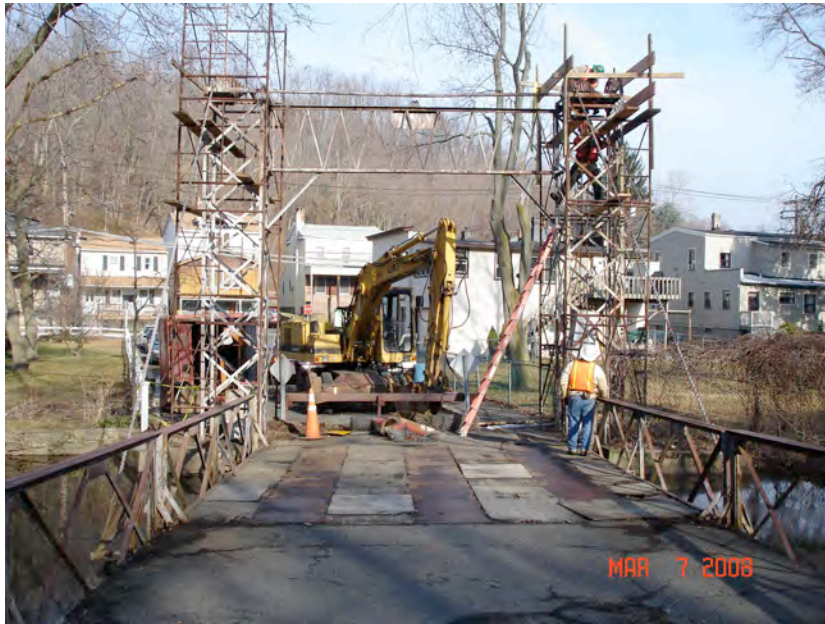
FIGURE 6: Demolition of steel towers
