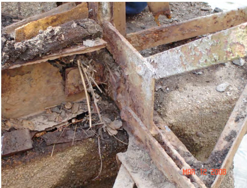
FIGURE 12: Severely corroded end floorbeam and truss gusset plate that were buried at the north abutment
