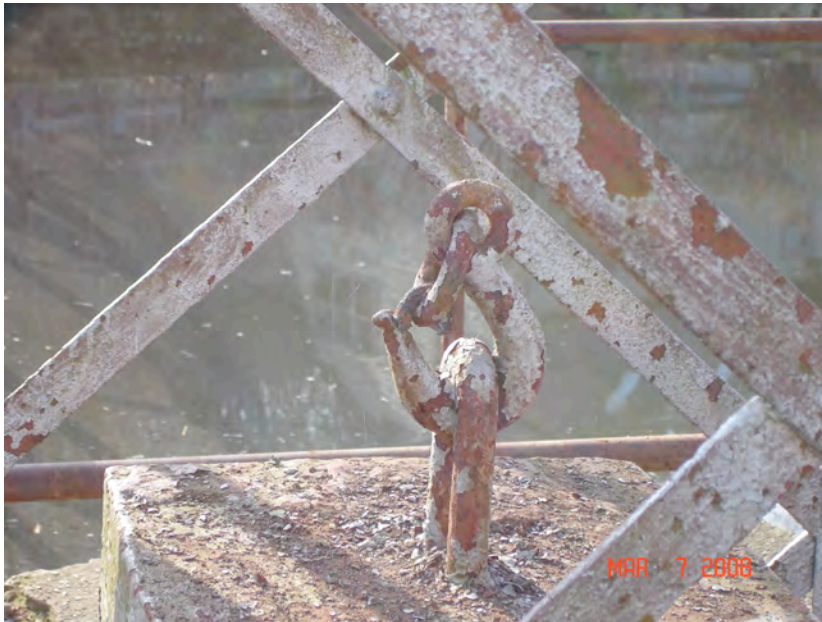
FIGURE 7: Severed link at northeast counterweight chain
