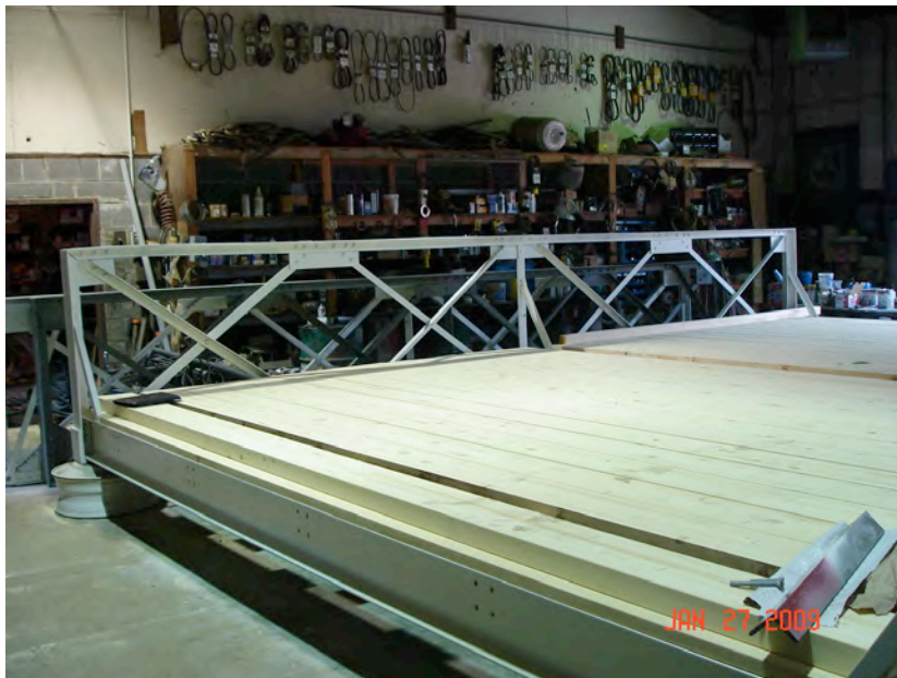
FIGURE 13: New timber deck and rehabilitated steel framing erected in shop
