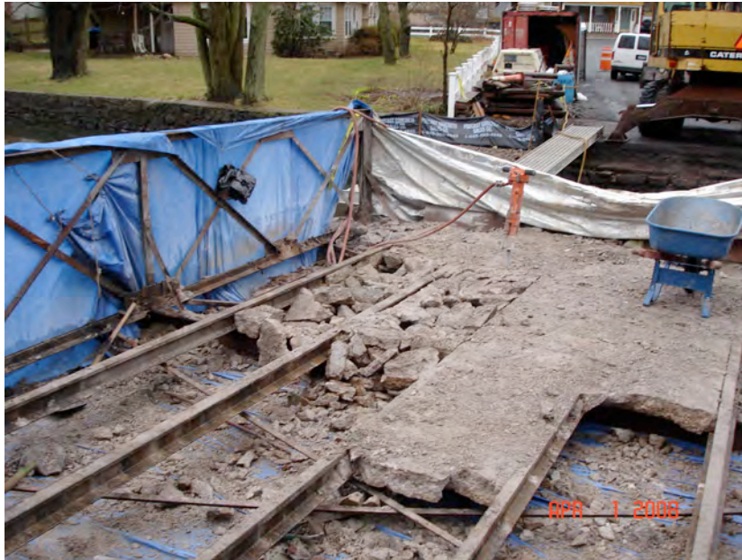
FIGURE 9: Demolition of the concrete approach deck uncovered used rails in the deck
