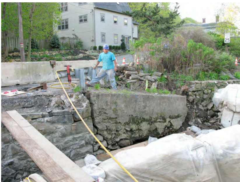
FIGURE 11: Movement of the Southwest Wingwall
