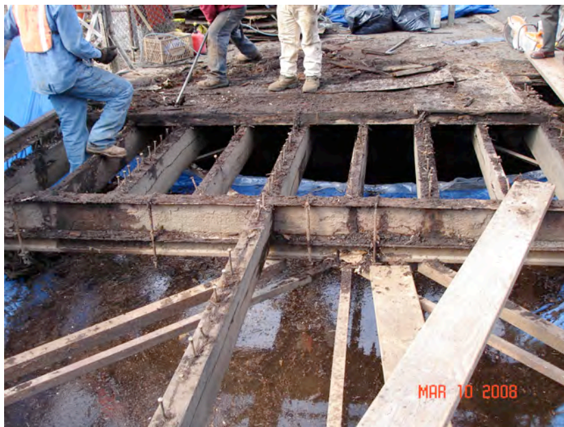
FIGURE 8: Demolition of timber deck
