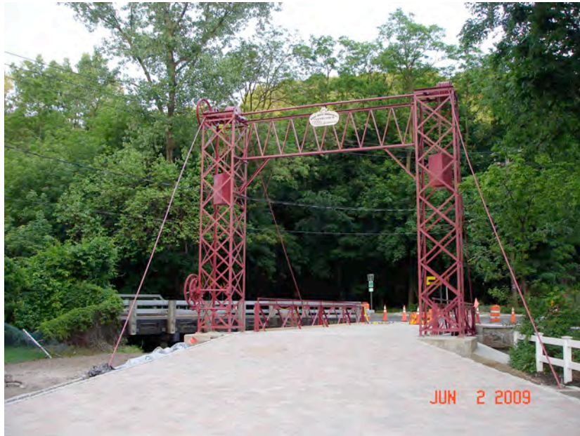
FIGURE 19: Substantial completion of the Bridge Street Bridge. Note the paving blocks used for the north approach
