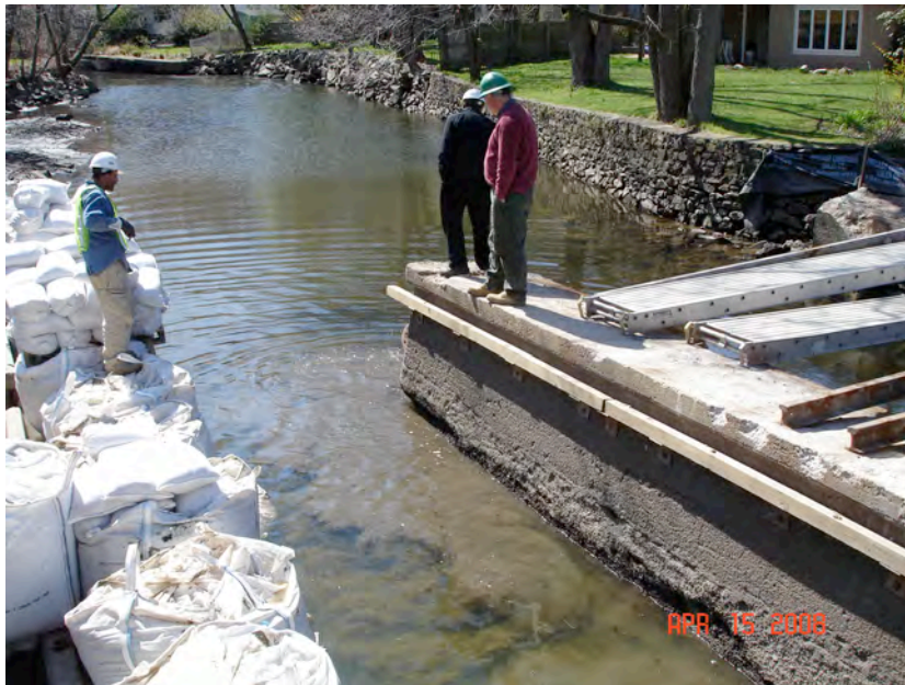
FIGURE 10: Concrete pier leaning toward the north
