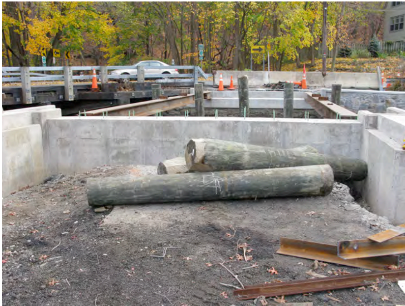
FIGURE 14: View looking south from behind the north abutment. Note new timber piers and the reconstructed southwest wingwall
