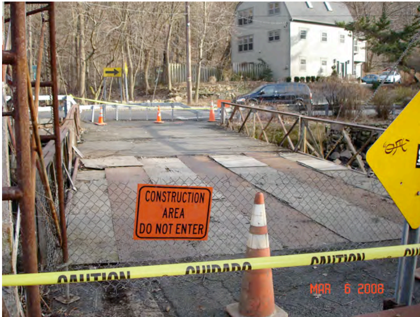
FIGURE 5: View looking South across the deteriorated timber deck on the bascule span at the start of construction. Also note the asphalt overlaid concrete approach deck and lateral deformation of the approach truss.
