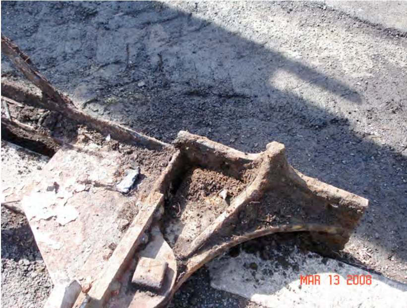
FIGURE 17: Existing movable bridge bearing uncovered during the removal of the existing draw span
