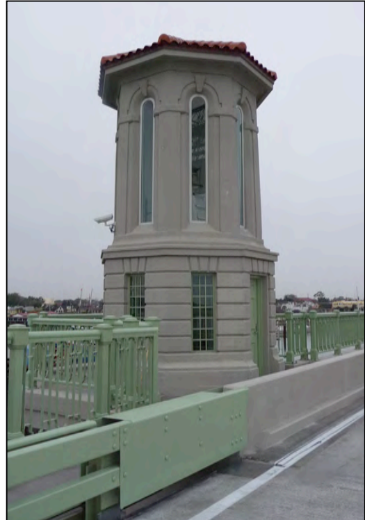
Figure 0 - Completed bascule pier tower. A coating that was color matched to the original bascule pier concrete was applied to all concrete surfaces above waterline for uniform appearance.
