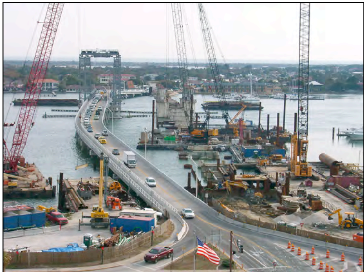
Figure 0 - Temporary bridge carrying traffic during rehabilitation.
