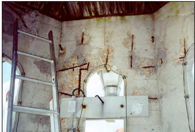
Figure 0 - Typical deterioration inside bascule pier towers.
