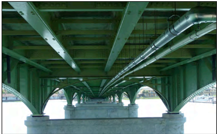
Figure 0 - New approach span framing. Note existing haunched girders re-used, modified to provide bearing support for the floorbeams over each pier.
