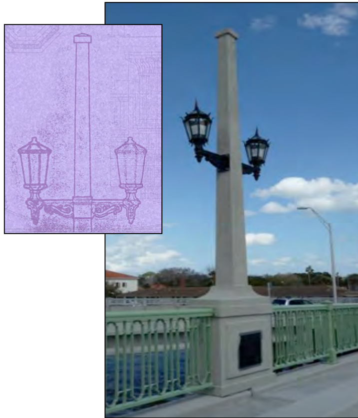
Figure 0 - Original design drawings detail for roadway lighting at left; replicated lighting at right.
