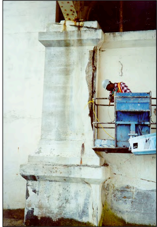
Figure 0 - Large spalls at bascule piers.
