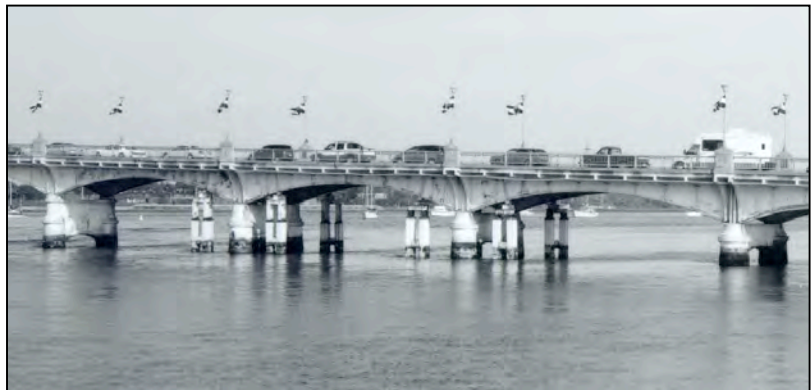
Figure 0 - Crutch bents to relieve loads at approach piers.
