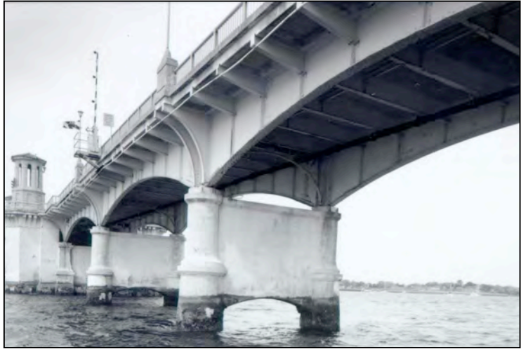
Figure 0 - Original haunched girder-floorbeam approach spans.
