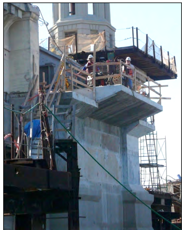
Figure 0 - Construction of new machinery platform at rear of bascule pier.
