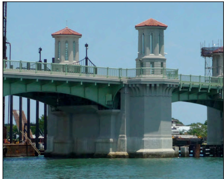
Figure 0 - Completed overlay containing impressed current cathodic protection system. Because of the size of the bascule piers, the addition of the overlay and build out of concrete cover did not affect overall appearance of pier.
