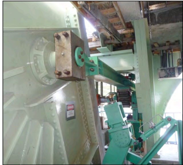
Figure 0 - View of strut attachment to rolling leaf.
