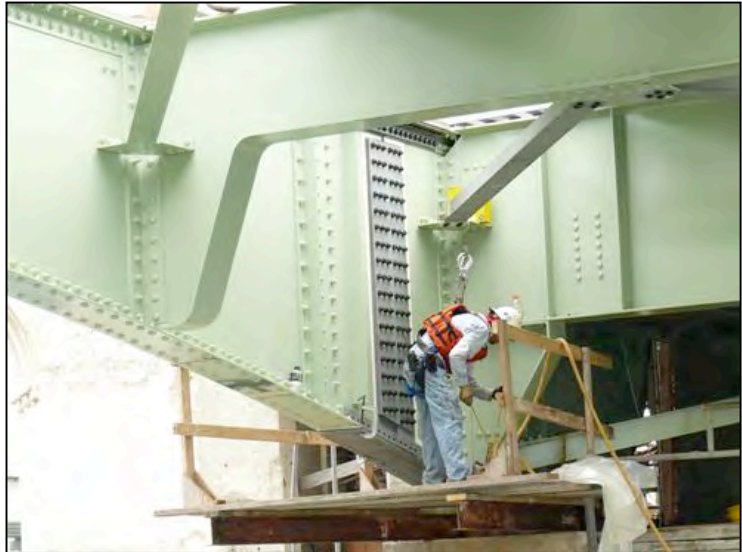
Figure 0 - New bascule span during construction. Note built up construction to left side of splice and built up welded construction to right and welded built up plate girder floorbeams.
