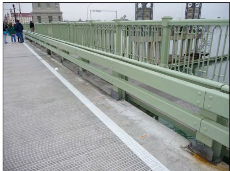
Figure 0 - New bascule span traffic barrier.
