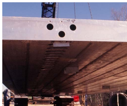
Little Buffalo Creek Bridge - US 58E (Shear studs on left and opening through which grout was pumped is on the right. Pictures taken in spring of 1997)
