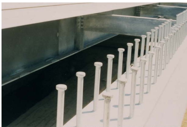
Little Buffalo Creek Bridge - US 58E (Shear studs on left and opening through which grout was pumped is on the right. Pictures taken in spring of 1997)
