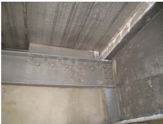
Little Buffalo Creek Bridge - US 58E illustrating the grout condition at the deck to girder connection. Pictures taken in March of 2011
