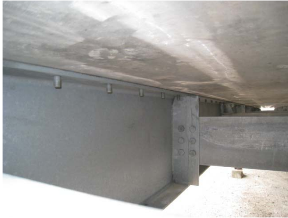
Slip Critical Connection using A-325 Bolts (Friction connections work with aluminum)
