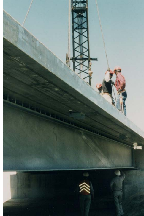
Little Buffalo Creek Bridge - US 58E (Center deck panel being positioned in left photo, deck to girder connection without grout in right photo. Pictures taken in spring of 1997)
