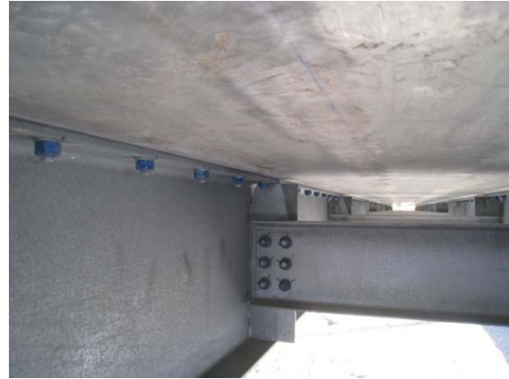
Slip Critical Connection using A-325 Bolts (Friction connections work with aluminum)
