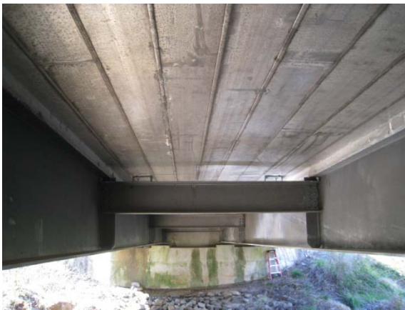
Little Buffalo Creek Bridge - US 58E illustrating the grout condition at the deck to girder connection. Pictures taken in March of 2011
