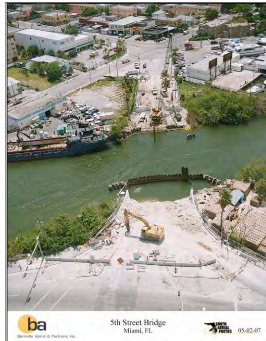
Demolition of Original Bridge
