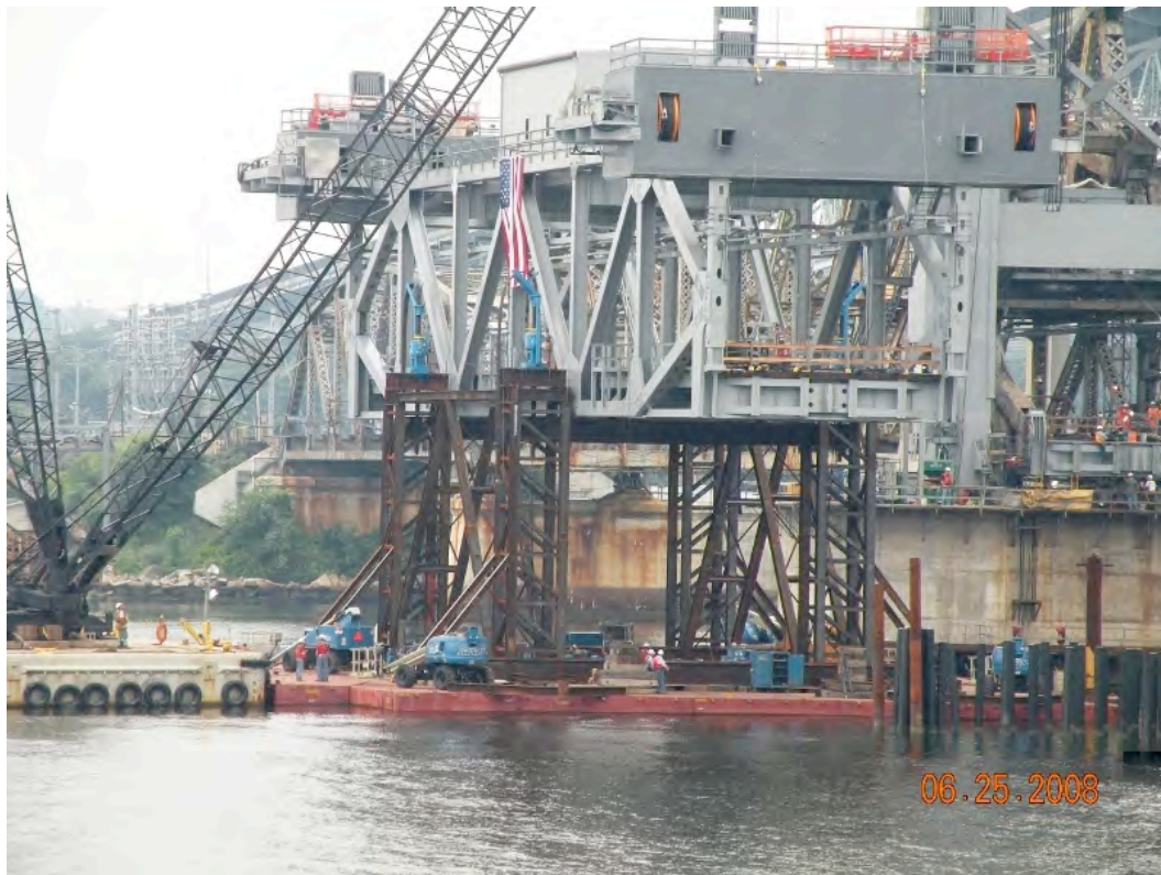
Figure 8 - Float-In of New Lift Span
