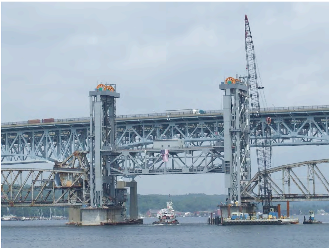
Figure 9 - Lift Span Partially Opened
