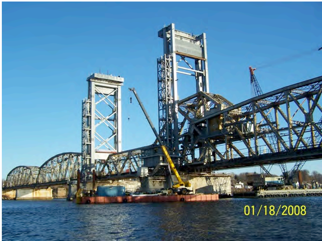
Figure 5 - Tower Steel Erection
