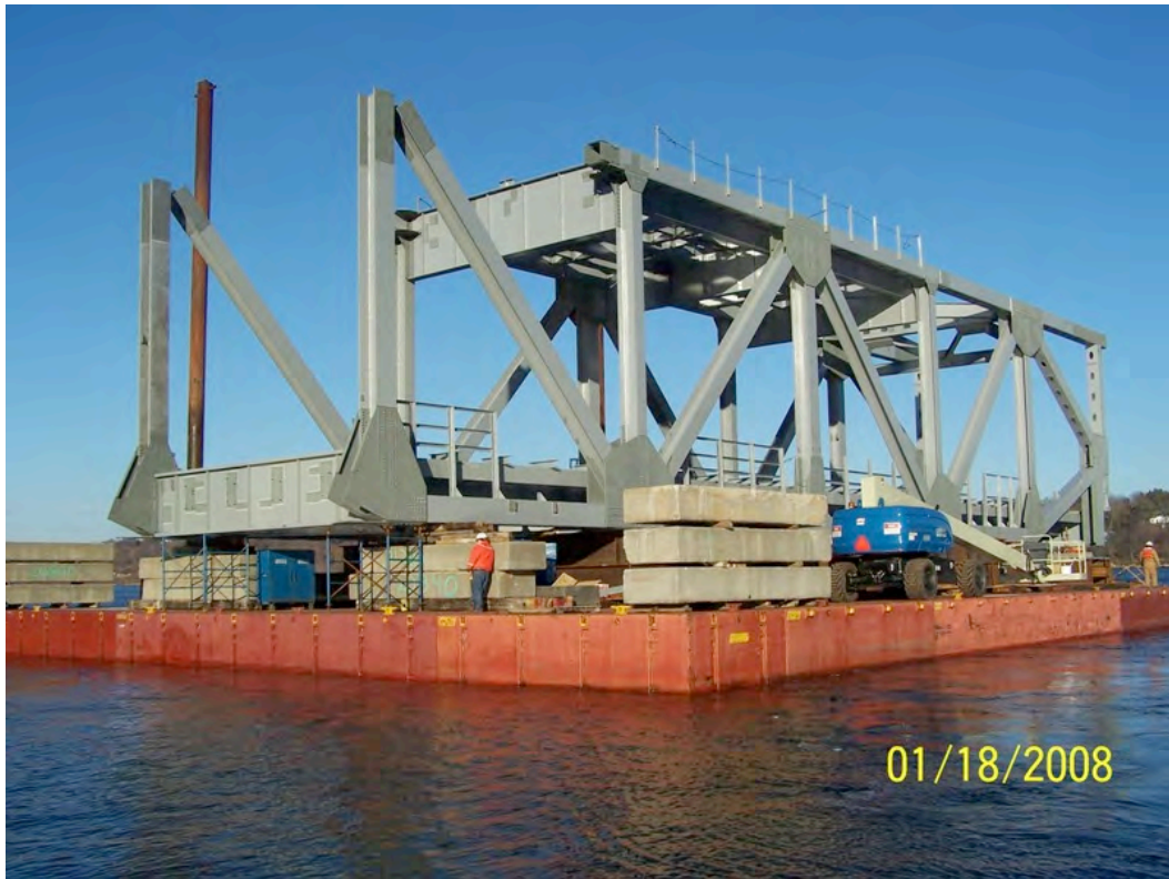
Figure 4 - Lift Span Erection
