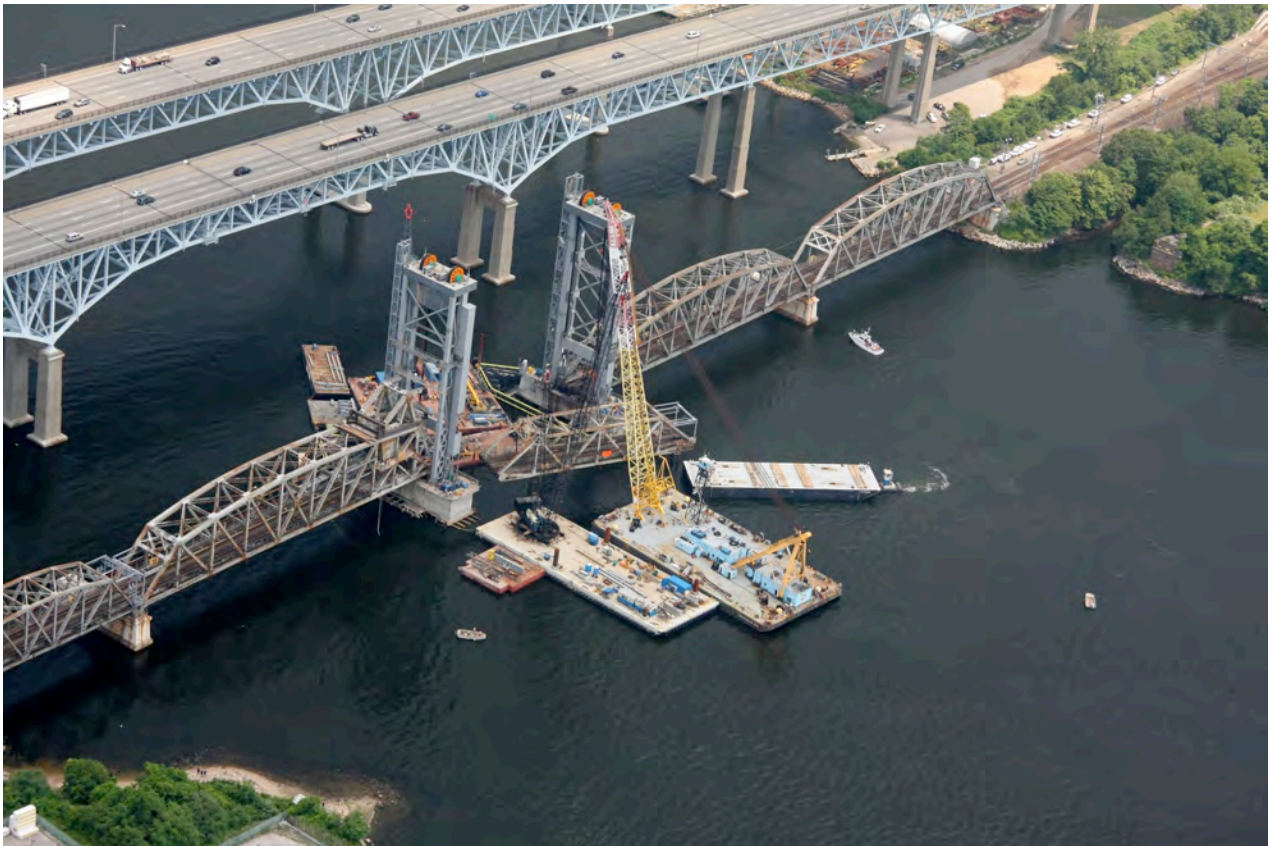
Figure 7 - Removal of Bascule Span C
