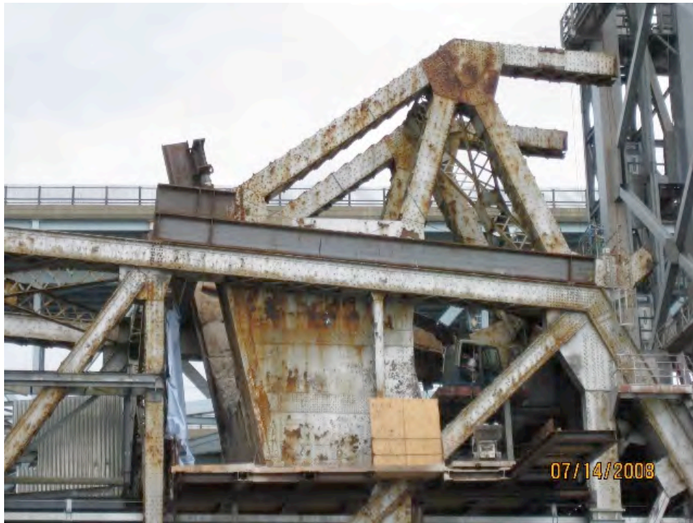
Figure 6 - Temporary Support of Existing Counterweight
