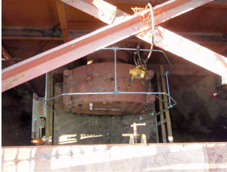
Photo 2: Typical Trunnion Bearing Assembly, Plan View
