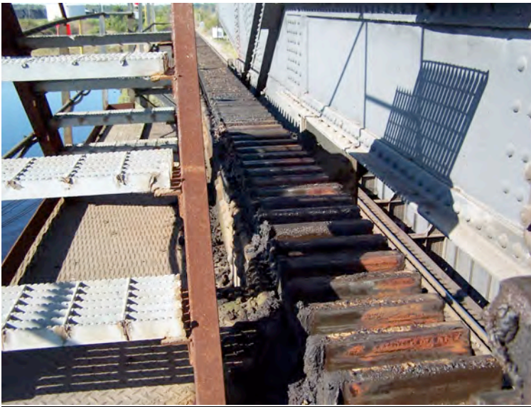
Photo No. 14: South rack looking west. Note: wear from tooth number 30 to the end of the rack indicating no contact between pinion and rack while closing.
