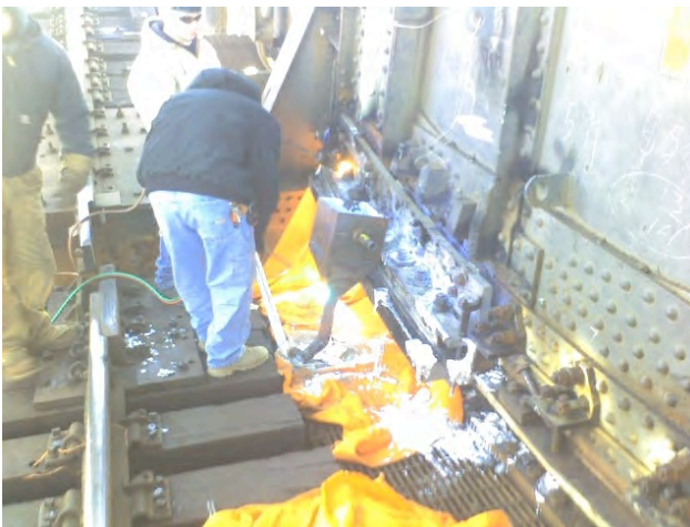
Photo No. 27: Installation of Segment 1. Pouring Zinc.
