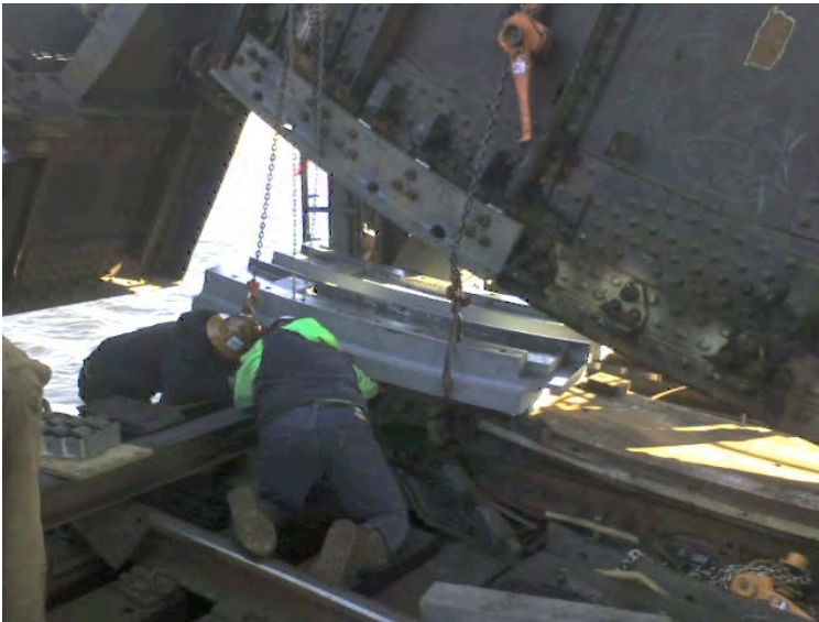
Photo No. 26: Installation of Segment 1. Note pre-installed flange angle.
