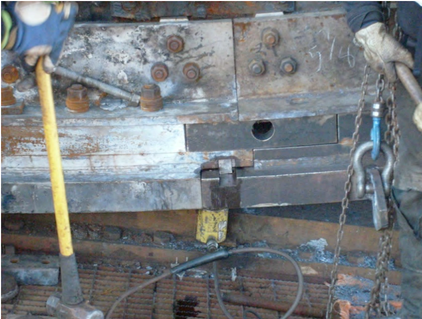
Photo No. 28: Installation of Segment 2. Note tongue and groove connection and fill hole for molten zinc in fill block.
