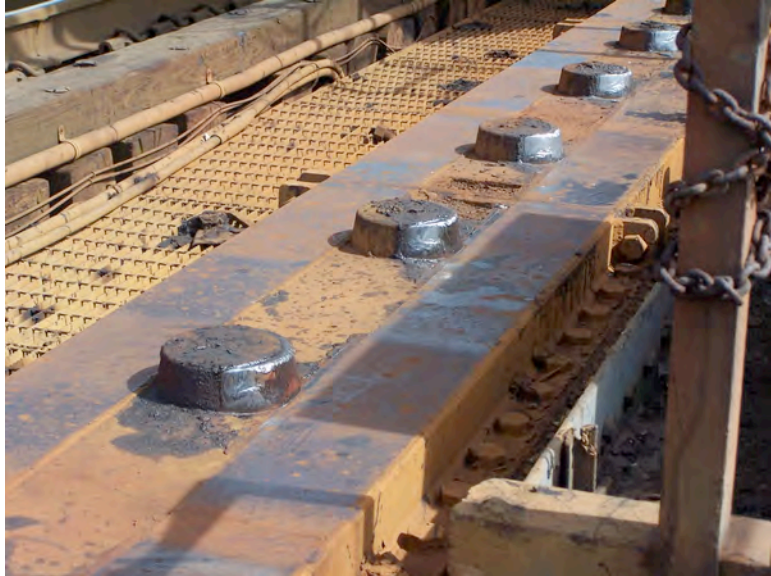
Photo No. 2: View looking northeast at the south segmental girder and flat track. Note shiny spots indicating wear of pintles.
