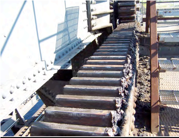
Photo No. 15: South rack looking east. Note: wear of rack teeth indicates contact between pinion and rack during opening.
