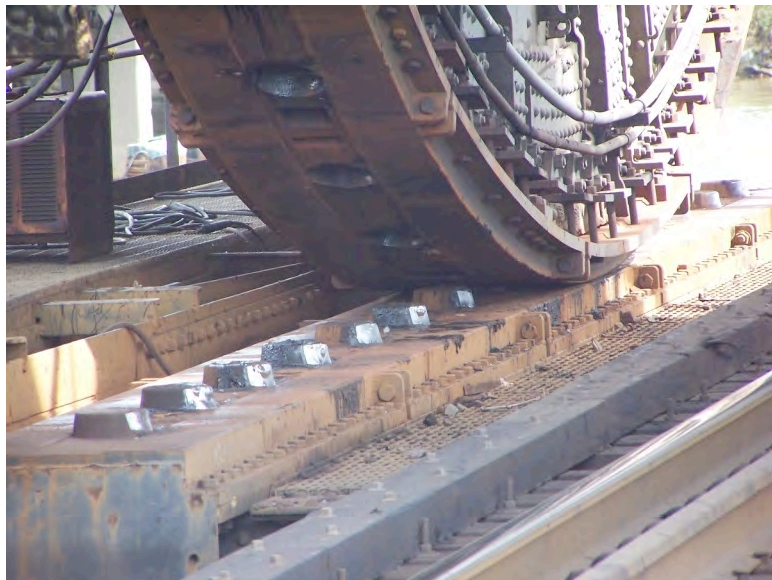
Photo No. 1: View looking northeast at the north segmental girder and flat track for Norfolk Southern Bridge 7. Note shiny spots indicating wear of pintles.
