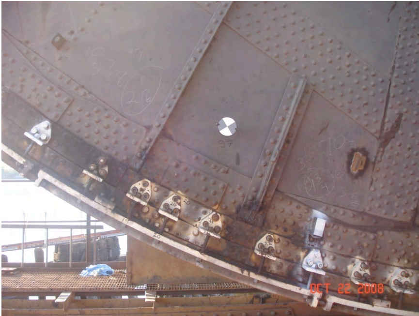
Photo No. 21: Survey Targets set up on the North face of the South Segmental Girder
