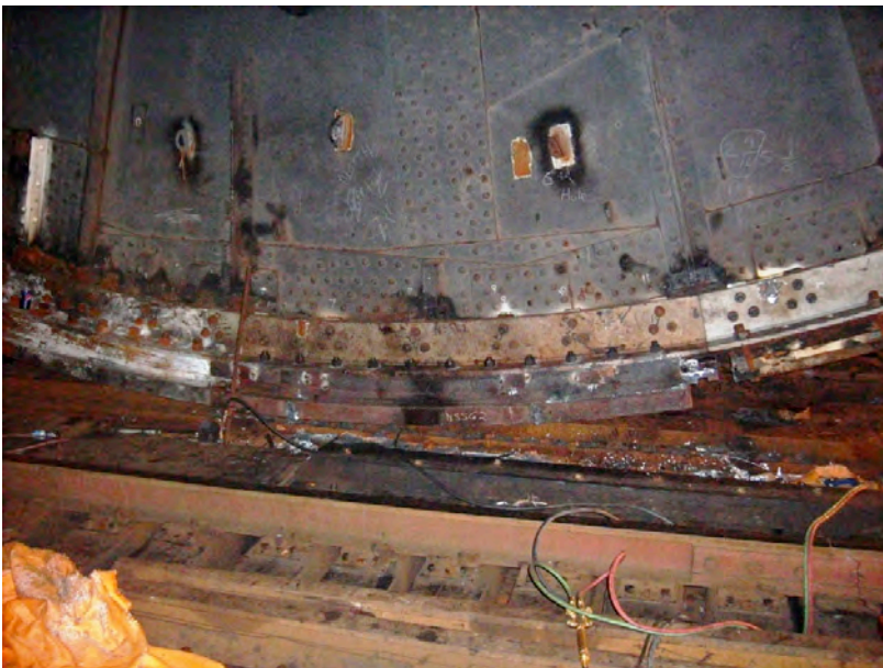
Photo No. 28: Installation of Segment 2. Note tongue and groove connection and fill hole for molten zinc in fill block.
